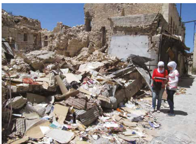
▲ DAMAGE ASSESSMENT AND DEBRIS MANAGEMENT IN THE ANCIENT CITY OF ALEPPO (SYRIAN ARAB REPUBLIC) © UNESCO/DGAM
