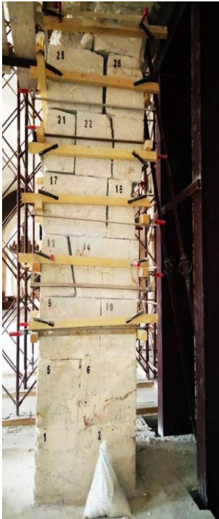
Documenting the column 205 before the dissemble
