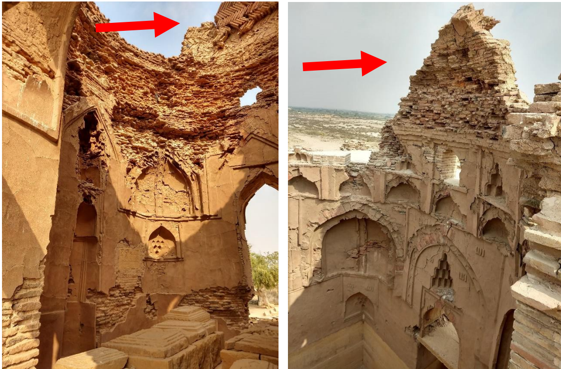
Figs. Sister Fatah-1 (l.) and Sultan Khos-1 (r.). Examples of fragile building fabric in danger of loss that require both regular monitoring and possible emergency stabilization to prevent collapse. Masonry dome remnants are particularly fragile because of the incomplete structure and their continued exposure to wind and rain. In these photos are also visible fragile areas of plaster and exposed masonry that require monitoring. Both of these monuments are also in need of drainage solutions for the interior spaces now exposed to the elements and possible location for pooling rainwater. ©J.Bell2019
