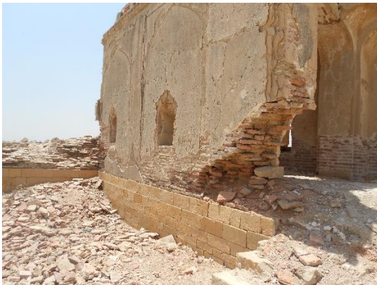
Figs. Lali-1 and Lali-2. Photos from before (2016, l.) and after (2019, r.) stabilization intervention. Brick masonry buttresses and infill masonry were added to stabilize the wall and prevent additional loss of materials. The Reactive Monitoring Mission highlighted that this intervention is effective as a temporary measure, but visually obtrusive due to its mass and negative impact on the form of the original structure. ©J.Bell2019
