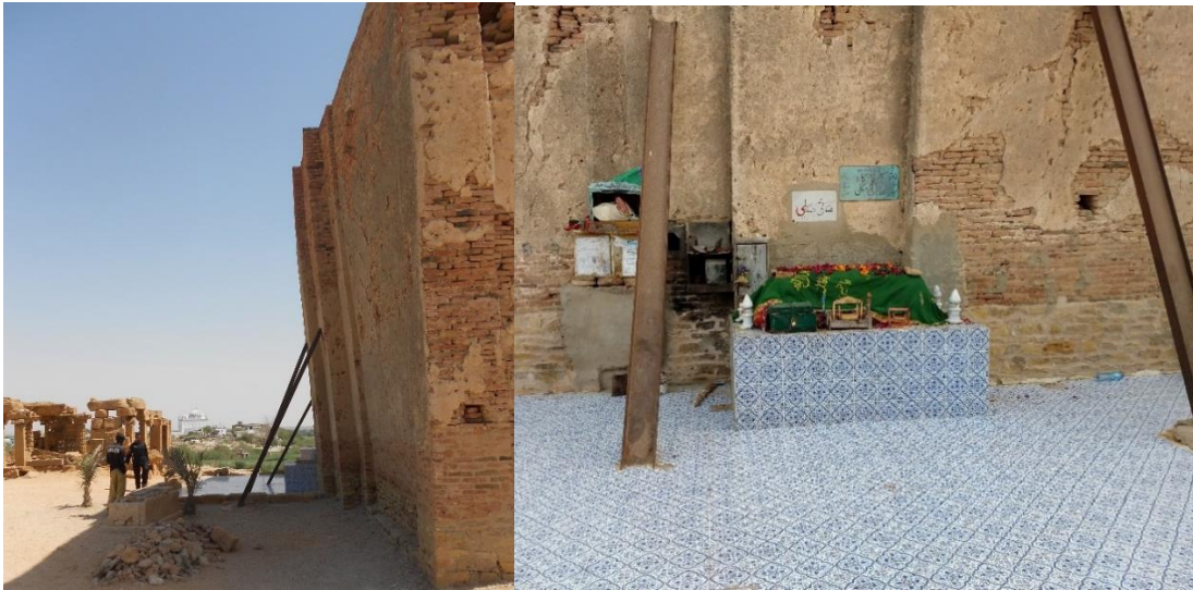
Figs. Jamia-3 and Jamia-4 (l. and r.). I-beams for stabilization in Jamia Masjid were put in place in the 1970s as temporary stabilization solutions. Although infill masonry has been added to the east side of the building as a structural intervention, there have been no efforts to monitor the effectiveness of the I-beams or to develop alternative, permanent stabilization solutions for the western portion of the structure. ©J.Bell2019
