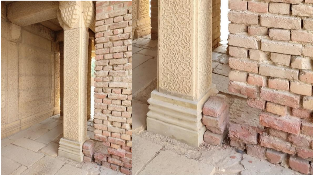
Figs. Issa Khan-1 and Issa Khan-2. Issa Khan Tarkhan II. Masonry pillars were constructed in the 1980s adjacent to original stone columns as stabilization efforts (l.). Although recent interventions on the roof and at the property aimed to address certain conditions of the monument, no effort was made to assess the condition of earlier structural interventions or develop more permanent solutions. A detail of one column (r.) shows that it has been undermined through loss of bricks. ©J.Bell2019
