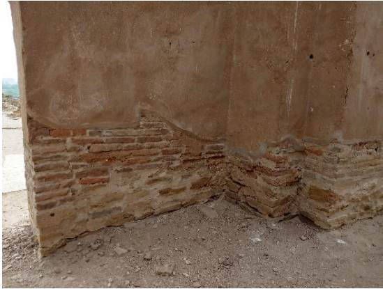
Figs. Jamia-1 and Jamia-2. Areas of infill masonry added to Jamia Masjid as stabilization measure (l. and r.). ©J.Bell2019
