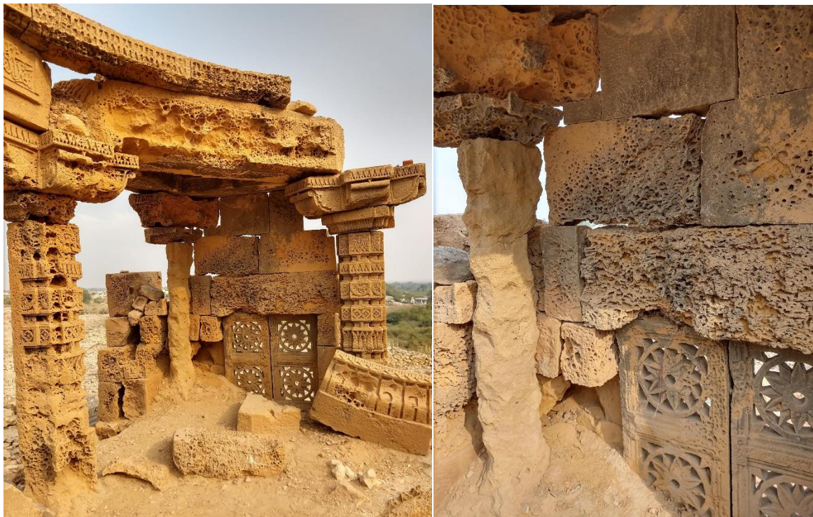
Figs. Madrasa-2 and Madrasa-3 (l. and r.). The advanced state of decay of the stones used in the monument have made it extremely fragile. Severely eroded stone elements are highly friable and those bearing loads of stones above are at risk of further damage that could ultimately lead to collapse of additional portions of the monument.
