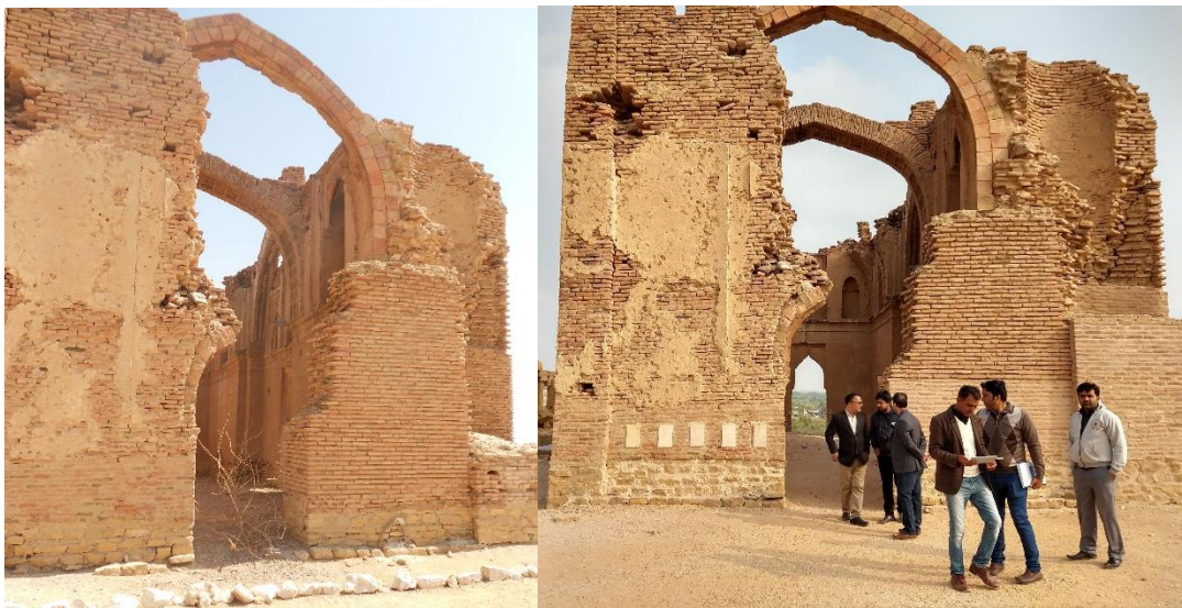
Figs. Jamia-1 and Jamia-2. South façade of Jamia Masjid in 2016 (l.) and 2019 (r.). Notice infill masonry on the right to address basal erosion and provide structural stabilization for the monument. A series of mortar/plaster tests are visible on the left with masonry repointing below.
