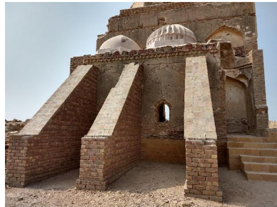
Figs. Lali-1 and Lali-2. Photos from before (2016, l.) and after (2019, r.) stabilization intervention. Brick masonry buttresses and infill masonry were added to stabilize the wall and prevent additional loss of materials. The Reactive Monitoring Mission highlighted that this intervention is effective as a temporary measure, but visually obtrusive due to its mass and negative impact on the form of the original structure. ©J.Bell2019
