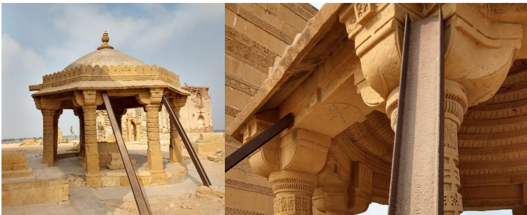
Figs. Tamachi-1 and Tamachi-2. The canopy of Jam Tamachi. Similar to Jamia Masjid, I-beams were used as temporary stabilization interventions in the 1970-80s (l.). It appears that the I-beams have caused damage to the fragile stone surface and continued lateral movement of the monument is causing the I-beams to become incised into the stone. Long-term stabilization interventions should be developed and implemented. ©J.Bell2019
