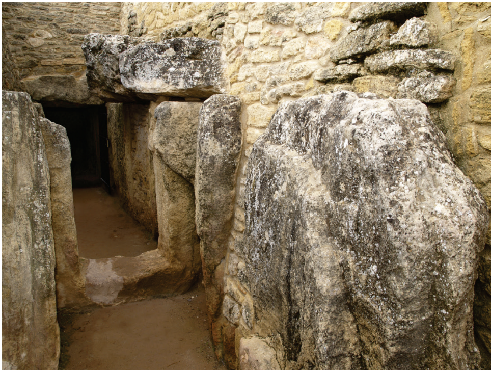
Perforated door in the Viera dolmen corridor
