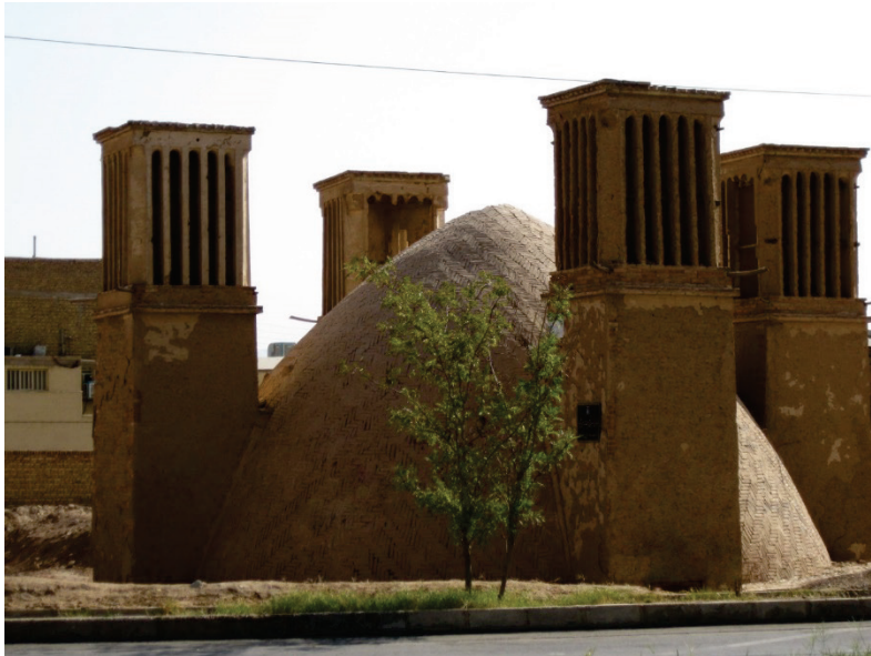
Hassan Ābād-e Moshir Qanat water reservoir
