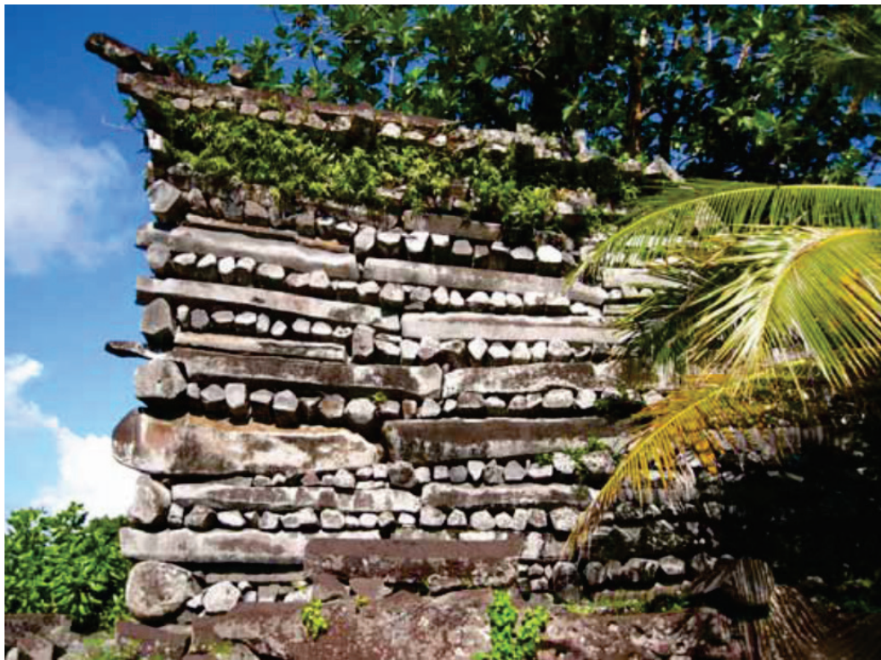
Columnar basalt built by in a header-stretcher technique, Nandowas Islet
