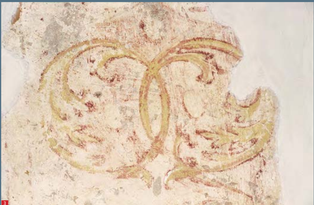
3 Detail of the northern fragment in the middle soffit arch of the west arcade, upper floor
