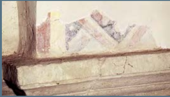
Beginning of a soffit on the north side, ground floor of the southern nave, eastern arcade Drawing of the find by Goege
