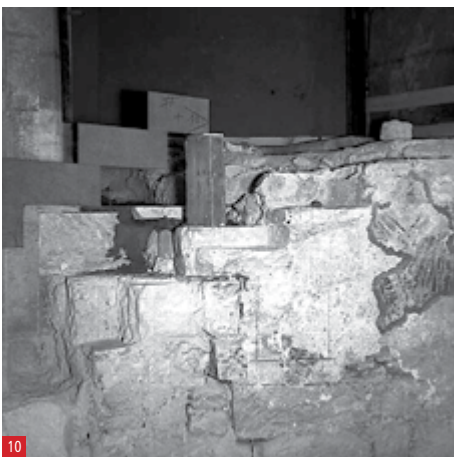
Saint-Denis, Carolingian choir, traces of the staircase on the northern wall (according to Formigé)
