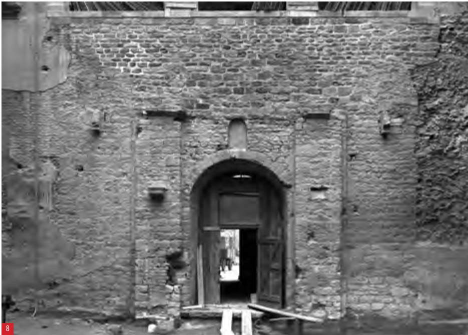
Minden, Cathedral, the eastern wall between the flanking towers of the westwork viewed from the east with the portal, the preserved wall projections of the central isle in the central room and the break-off traces of the wall projection between the central room and the northern isle in 1950
