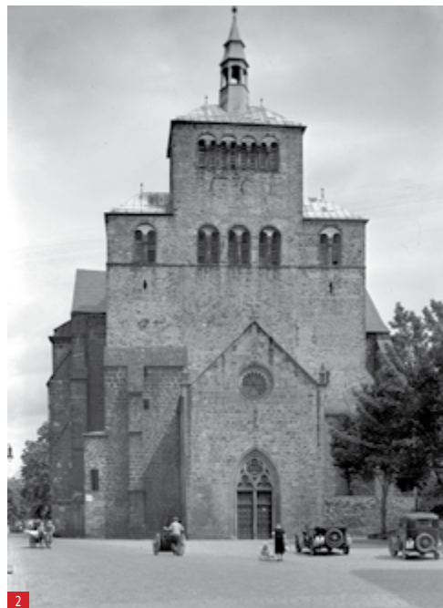
The Minden Cathedral viewed from the west prior to WW II
