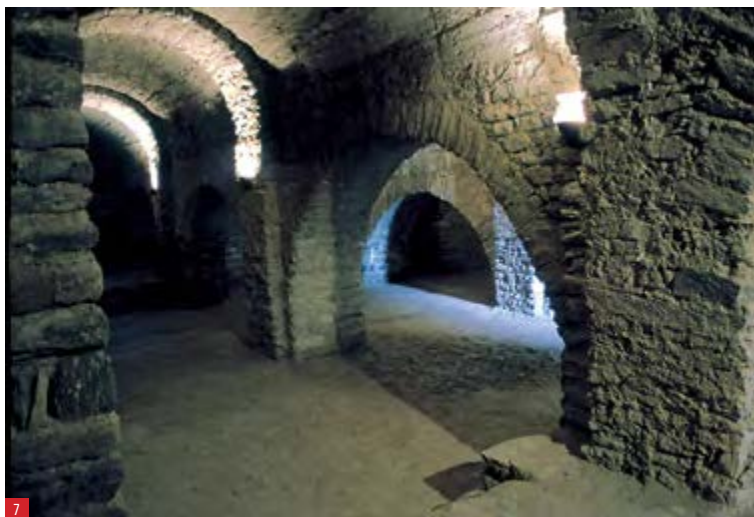
Saint-Michel de Cuxa, abbey, barrel vault of the pre-Romanesque crypt (A. Hartmann-Virnich)
