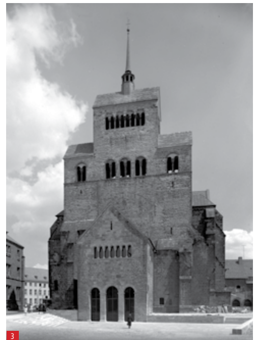
The Minden Cathedral viewed from the west after the reconstruction
