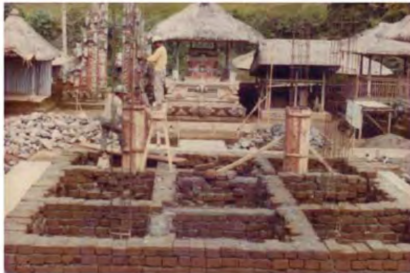
Restoration Work in the Temple, 1983
