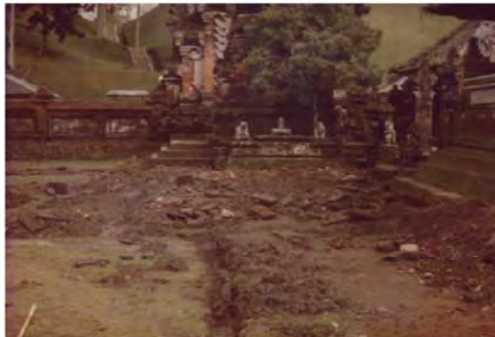
Condition of Tirtha Empul After Earthquake Disaster, 1972
