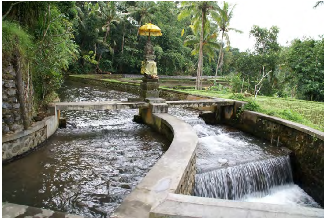
The main irrigation canal from the spring at Tirtha Empul, branching into flows for Pulagan and Kulub Atas
