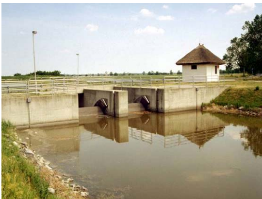
Sluice on the Einser Canal
