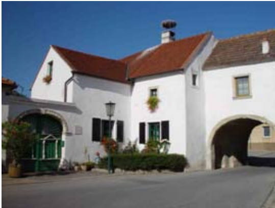
Town gate at Purbach
