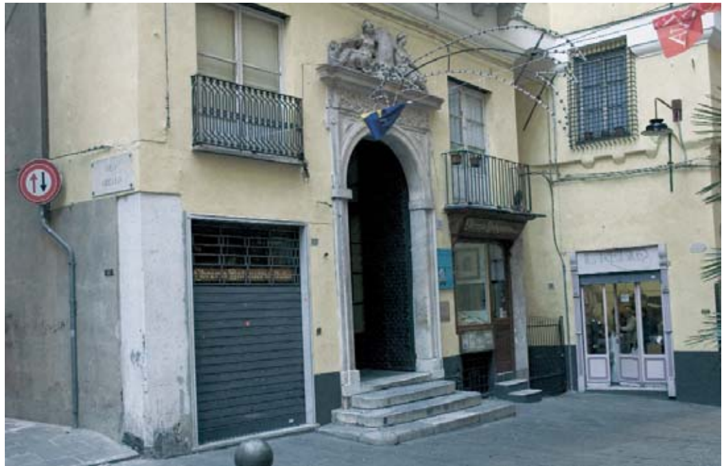
detail of the main façade
