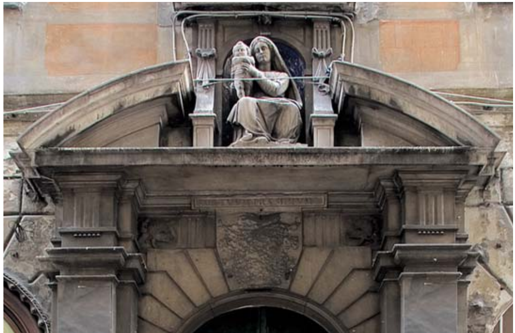
detail of the doorway
