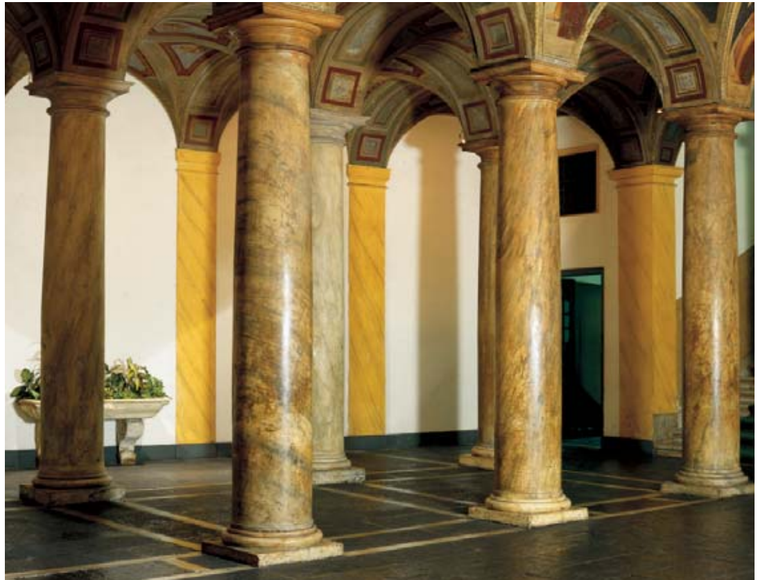
atrium with columns
