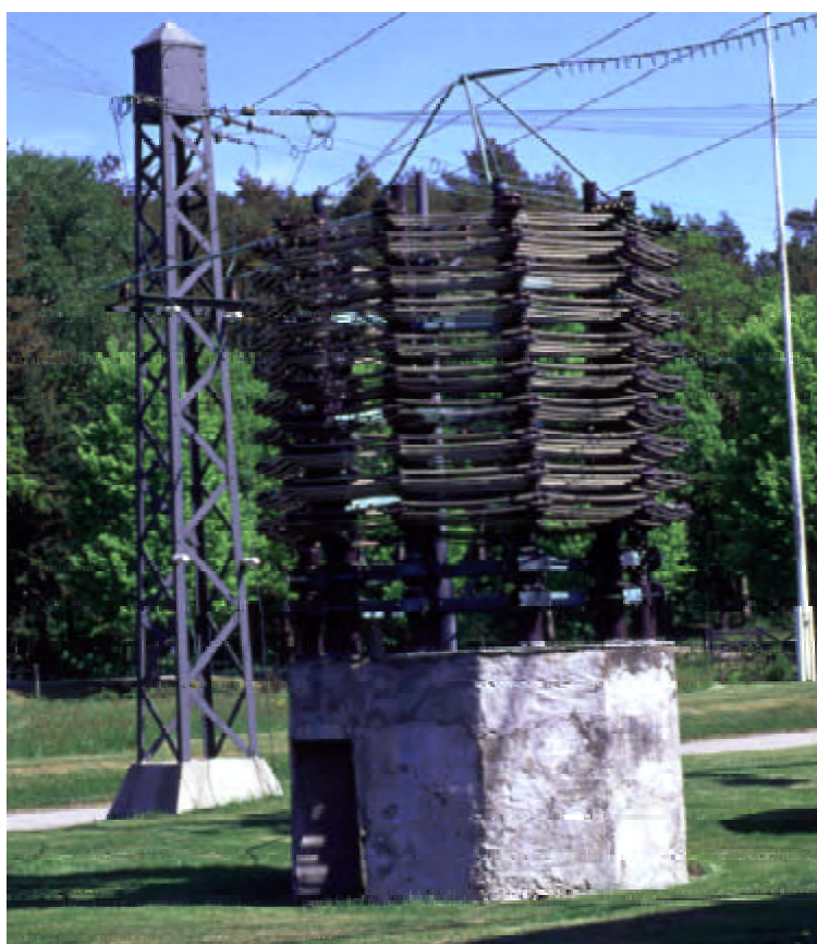
Tuning coil at feeder end, 2000
