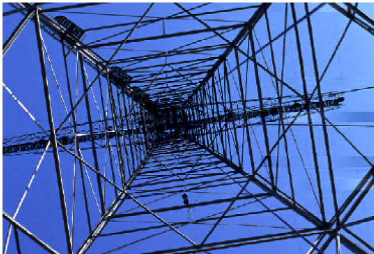
Detail of a tower, 2000
