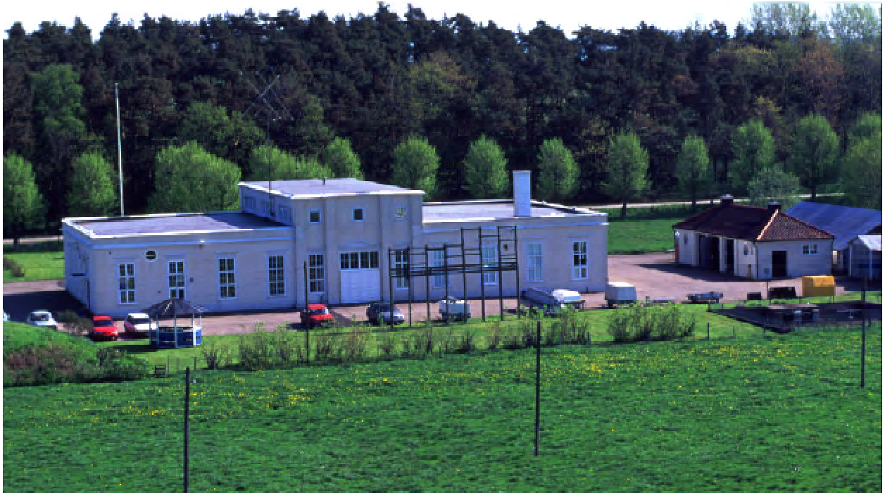
Transmitter building, 2000. The station garage is seen to the right.
