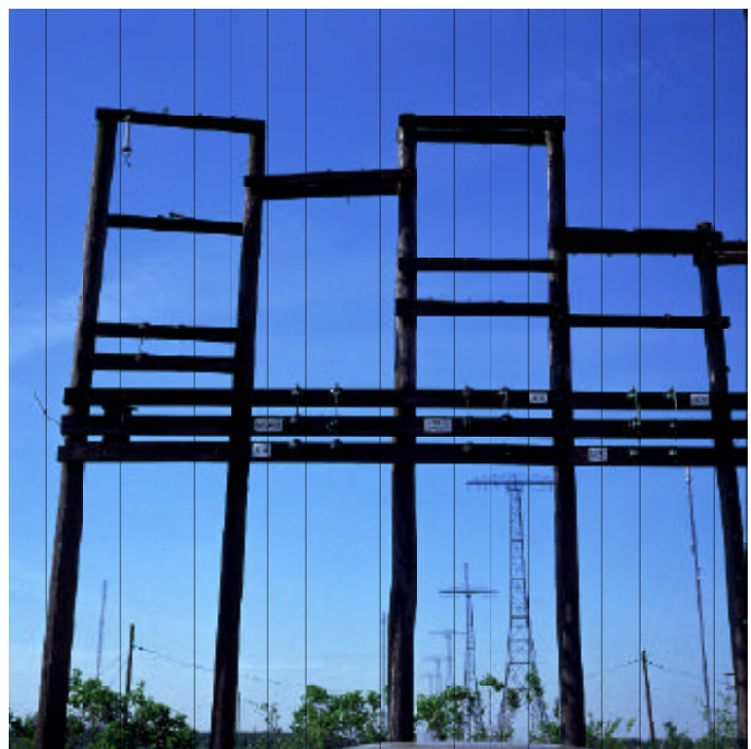
Remnants of switching rack for shortwave rhombic antennas, 2000
