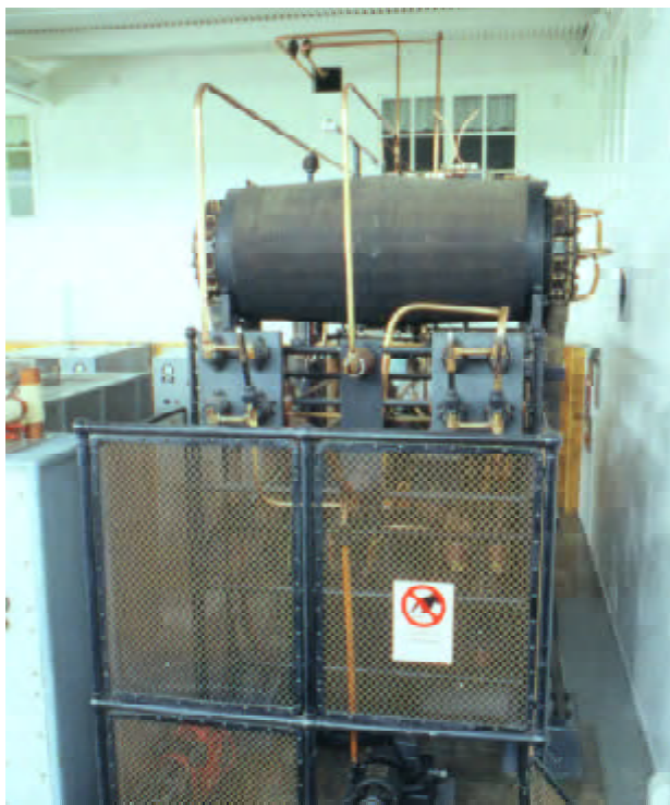
Radio-frequency rack 2001. Radio-frequency power transformers on top of the rack, magnetic amplifiers on the floor, capacitors to tune amplifiers on shelves. Photo: Bengt Spade
