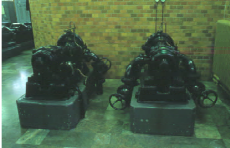
Cooling-water pumps, 2001
