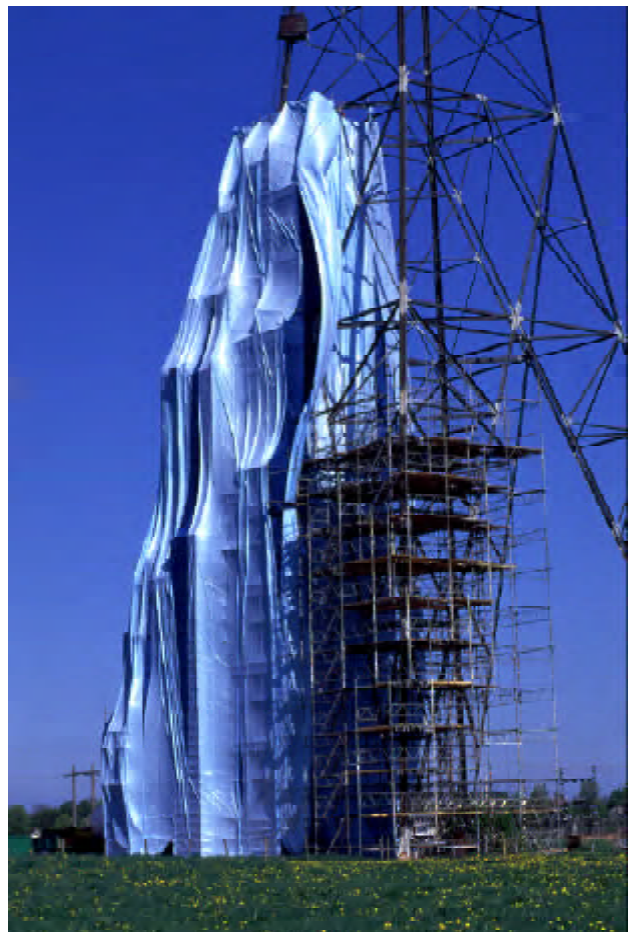
Repainting of antenna tower, 2000 Photo: The Museum in Varberg, Arne Persson
