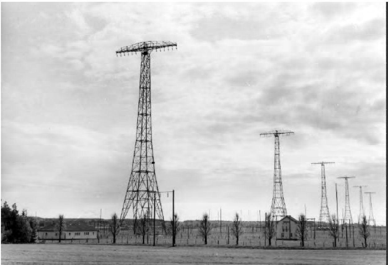
The antenna plant with its six towers
