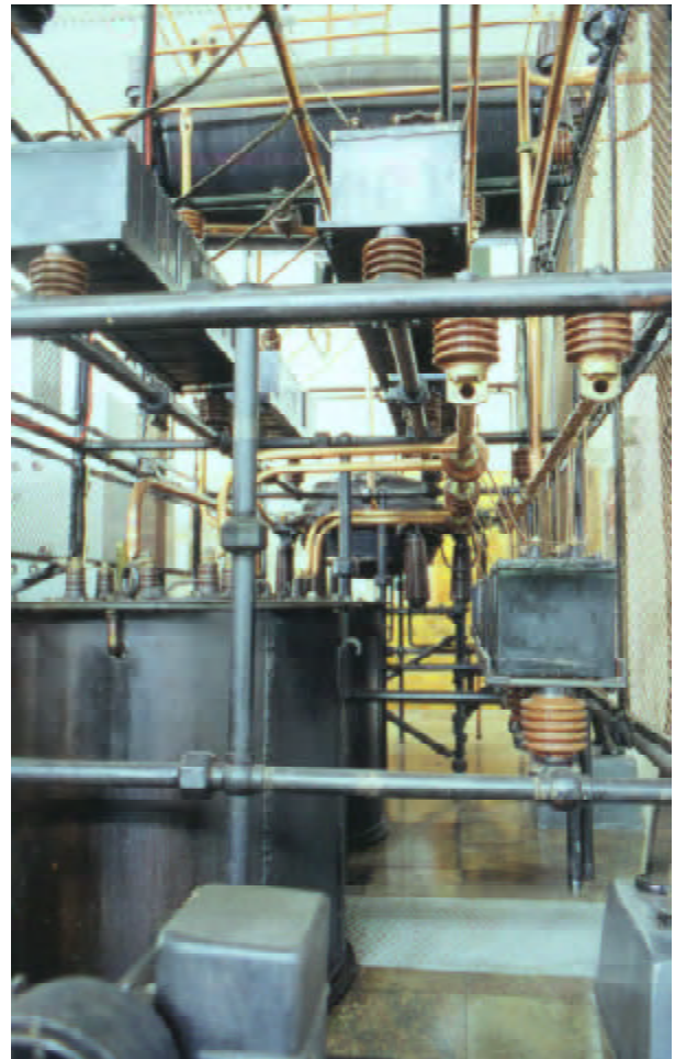
Detail of radio-frequency rack, showing the magnetic amplifiers, 2001. Photo: Bengt Spade
