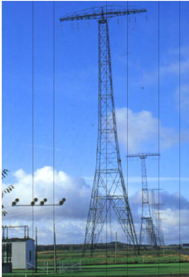
The antenna plant and ice-melting transformer house, 2001
