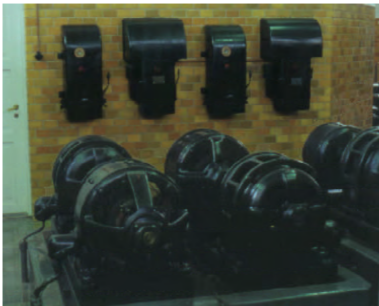
Motor generators, 500V, 2001
