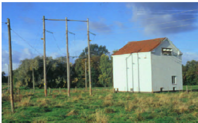
Mains transformer building, 2001
