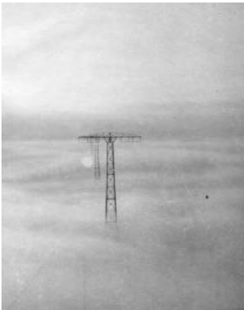
The antenna towers project above the fog, c 1925
