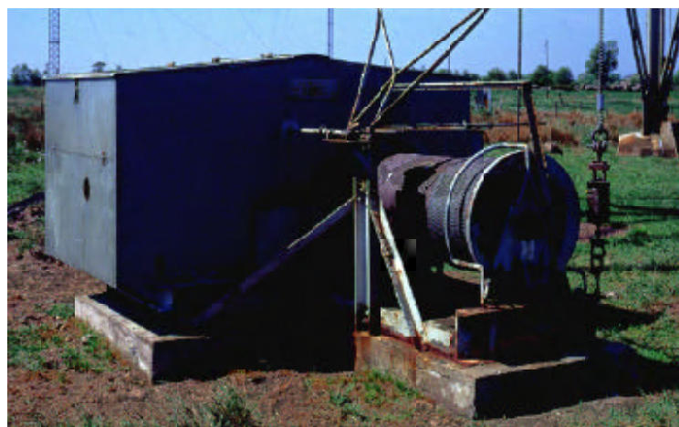
Hoist for lift basket of an antenna tower, 2000
