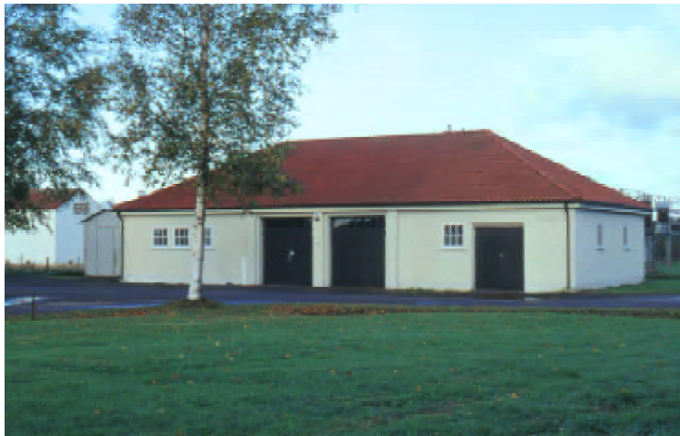
The station stores building, 2001
