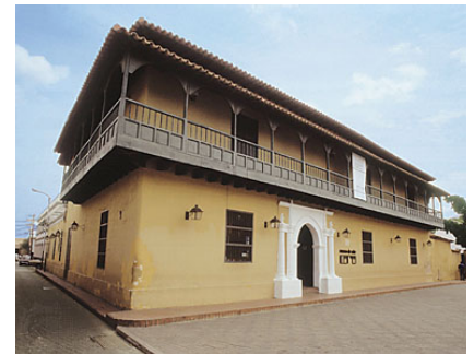
Supported balconies which canbe considered a variant of the brace, with splashboard of small roof on straight feet of wood, a very used solution in South America
