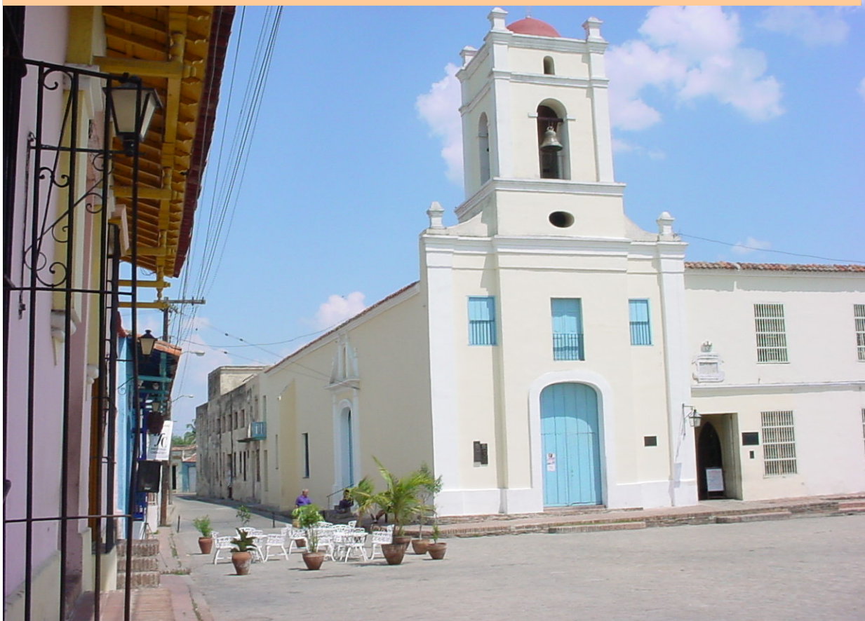
Rehabilitation of the Provincial Center of Patrimony. Arq. Ma. Herminia Olivera Hernández, 1987
