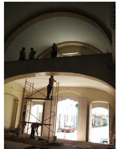
Works of rehabilitation in El Carmen church.
