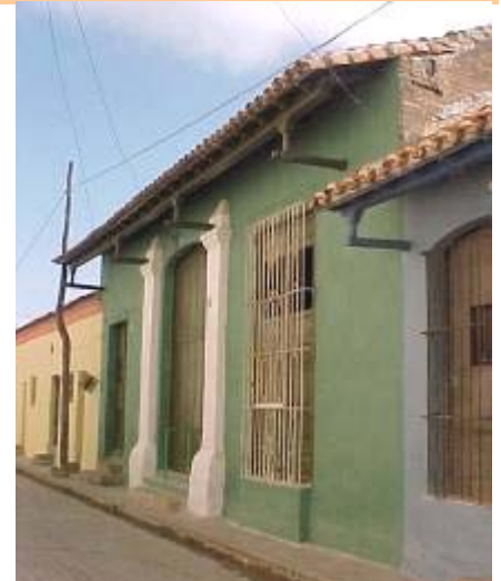
Eaves, rowlocks, penthouses and principally those of braces, which are originally from Camagüey
