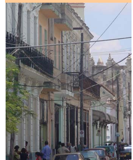
Most of electric and communicative nets is air.
