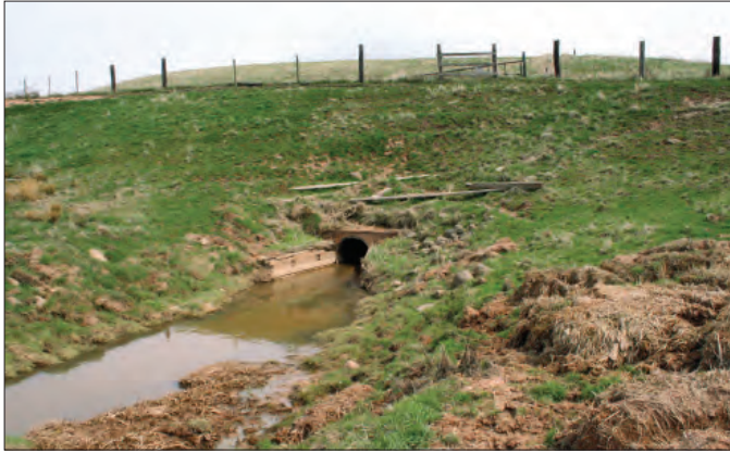
2-6 A working aboiteau drains water from the dykelands.
