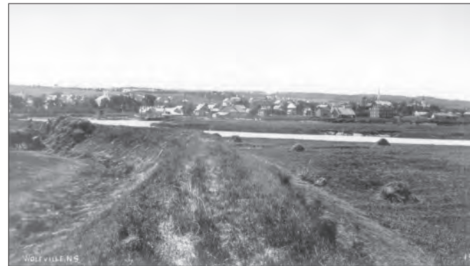
2-52 During the 1940s, federal and provincial governments launched programs to repair and rebuild dykes in the maritime provinces, including these at Grand Pré.
