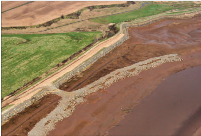
5-4 Breakwaters and rock facing on dykes mitigate the impact of storm surges.
