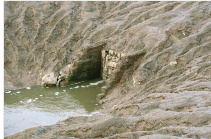
3-15 Modern aboiteaux use the same design and updated materials as those first constructed in Grand Pré by the Acadians.
