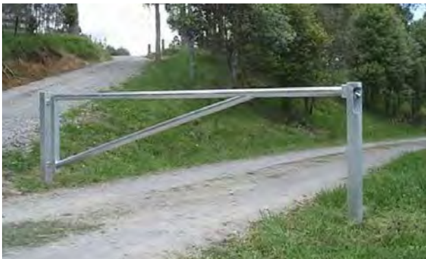
Illustration 17: A simple gate structure signage will further discourage access.
