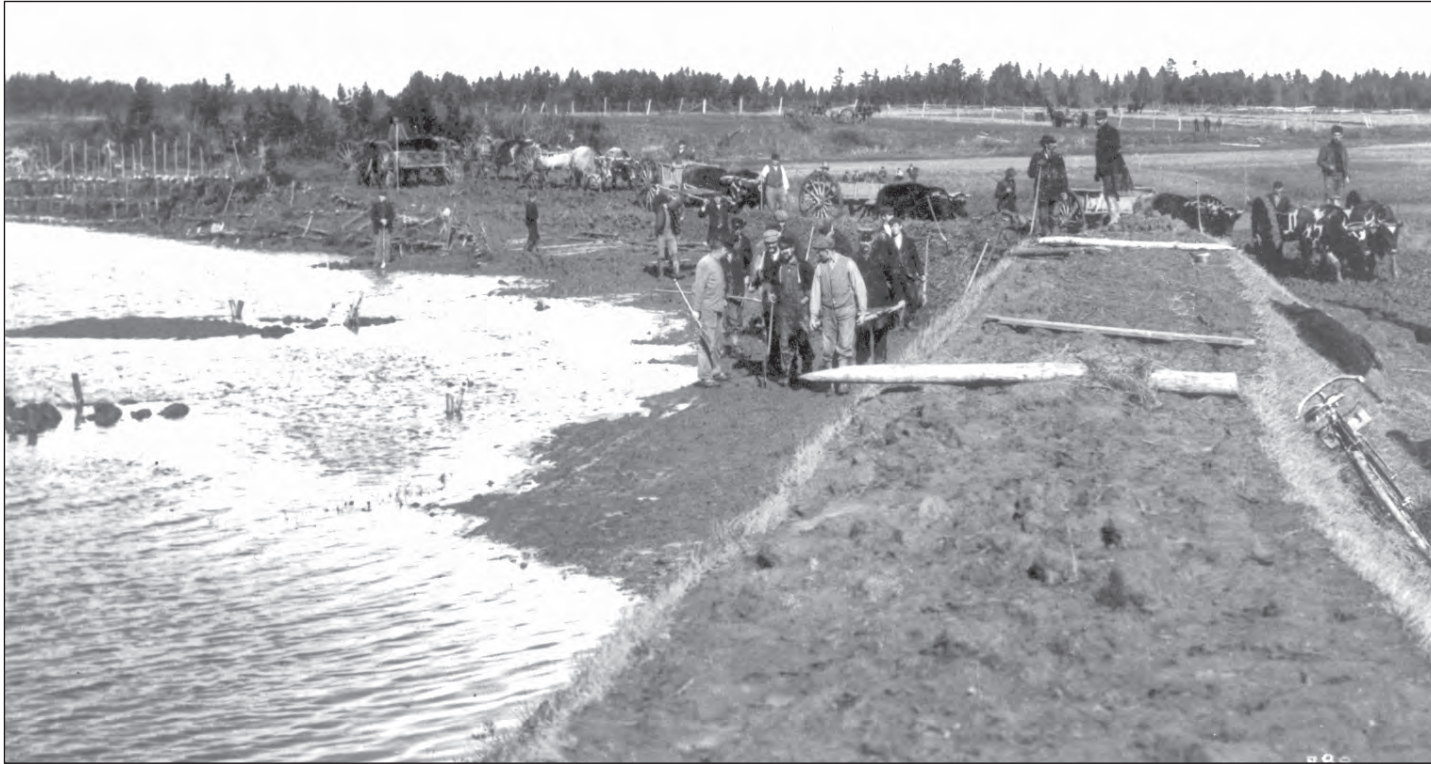
2-36 Repairing the dykes at Grand Pré, circa 1900. The tradition of building and maintaining dykelands collectively began with the Acadians and continued with the New England Planters and successive generations of farmers.
