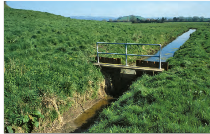
3–5 The tidal doors at the Gwent Levels (United Kingdom) allow water to leave the reclaimed land.
