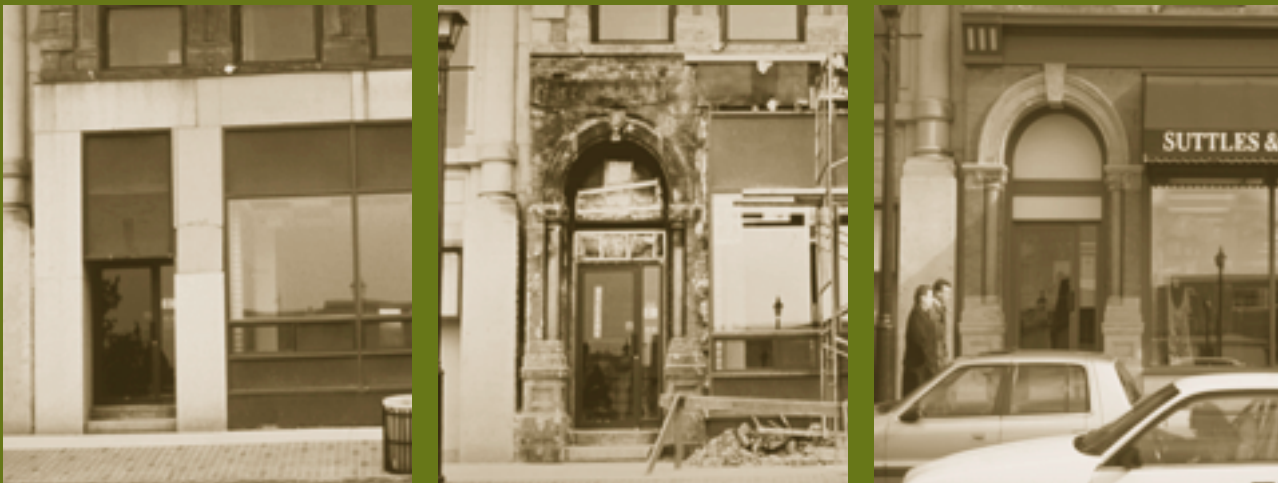
Restoration of a storefront may involve removing inappropriate cladding dating from a later period. Recreating a missing feature, such as the awnings on this storefront in New Brunswick, should be based on physical or documentary evidence.
