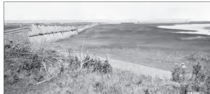
3-24 & 3-25 Dykes in Grand Pré are still topped with vegetation from the salt marshes. Rock facing is currently used to help withstand the force of the tides, rather than the wooden plank facing that was common in the 19th century.
