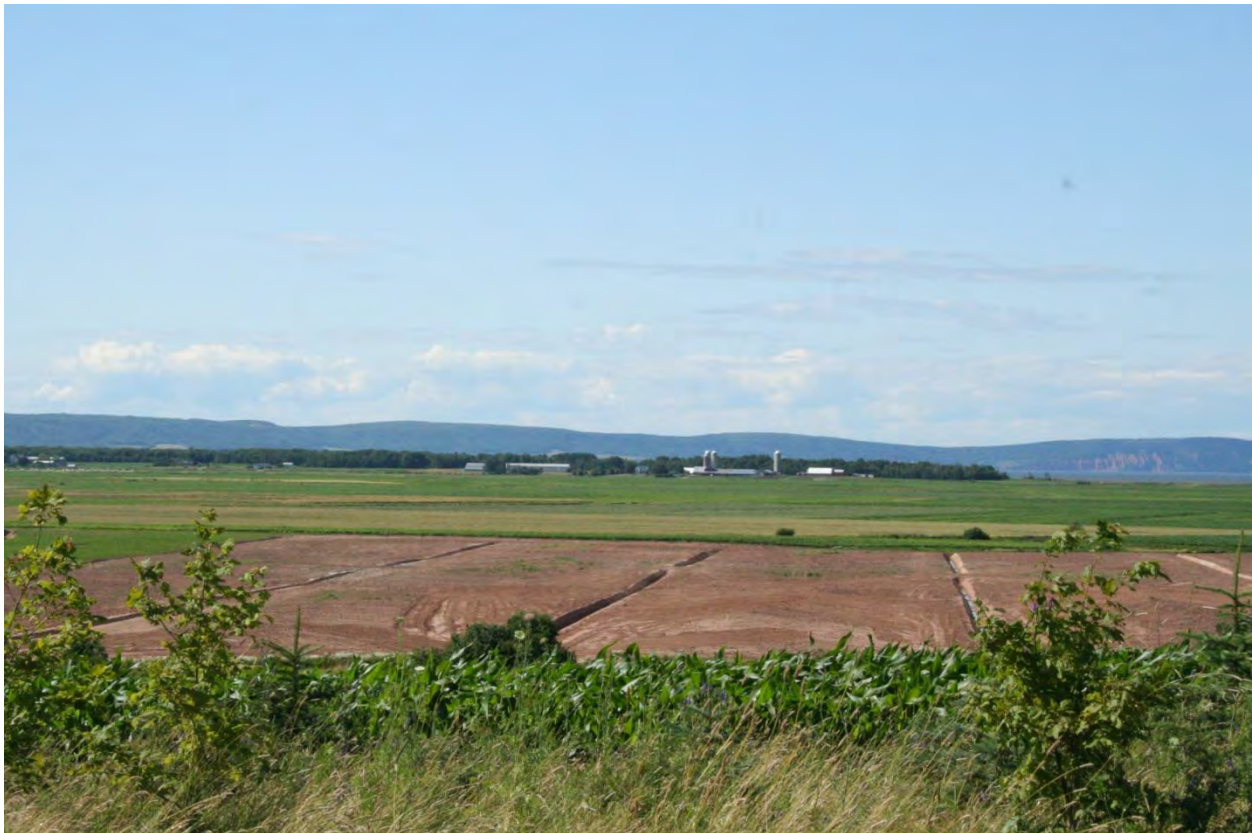
Figure 15: Drainage work on a field in Hortonville.
