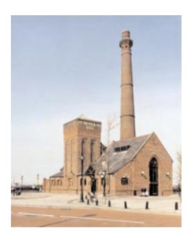
Little is known, and nothing survives, of the hydraulic power supply to the warehouses prior to modernisation of the system by G. F. Lyster, Hartley's successor, in the late 1870s. This 1878 pumphouse is in the characteristically elaborate mixture of common brick, pressed brick, sandstone and terra-cotta favoured by Lyster, but probably designed as an 'add-on' to the structure of the building by Arthur Berrington, the long-serving architectural draughtsman in the Dock Yard.
