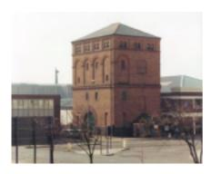
The Pumping Station was built to service the railway tunnel underneath the Mersey. Built of common brick with blue and red brick dressings, it has the restrained classical decoration frequently found on late Victorian utility structures.
