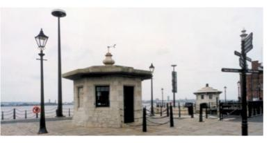
These little buildings are a tour de force of masonry construction. Hartley's technique of building in random granite (part ashlar, part dressed rubble) was extremely durable, but also cheap and this "Cyclopean" form of construction is an ancient form of masonry, in which the irregular shaped stones, from immense to minute size are assembled with very fine joints and a flat surface.
