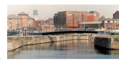
The later half-tide dock is faced in granite. At only six metres or so wide, Duke's Dock is relatively narrow compared to all of the other remaining docks and appears more like a canal than a dock. However, it should not be overlooked as it has the most complete 18th century dock retaining walls in Liverpool.
