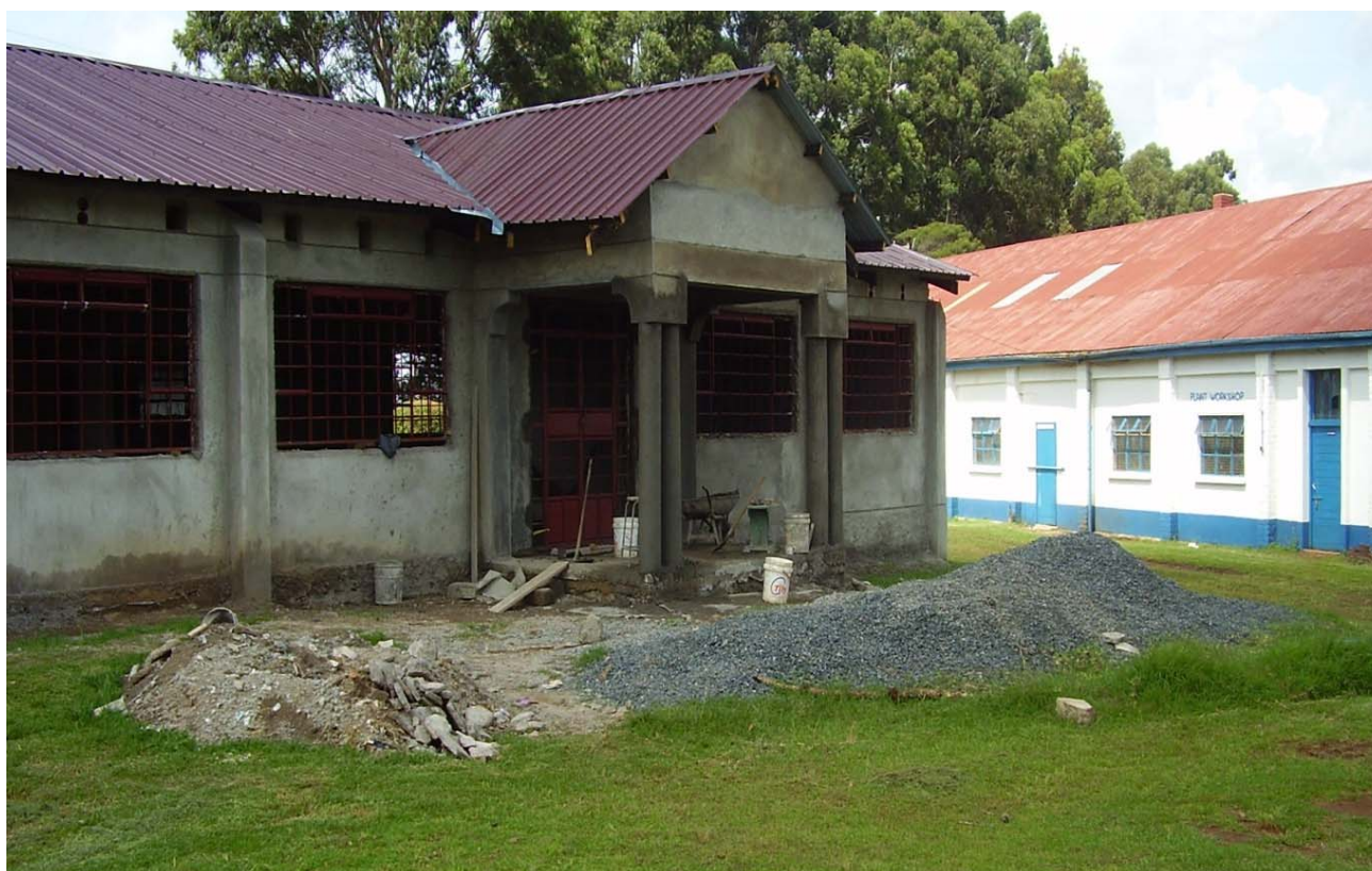
Figure 9: The new library under construction
