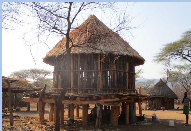
The Tonga of the Gwembe valley build elevated sleeping quarters known as Ingazi, made of poles and situated away from other houses in the homestead. They help reduce the spread of disease by ensuring physical distancing while providing safe quarters for the patients.
