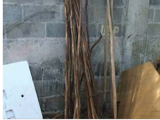
Photo 54 Guava poles used as reinforcement
