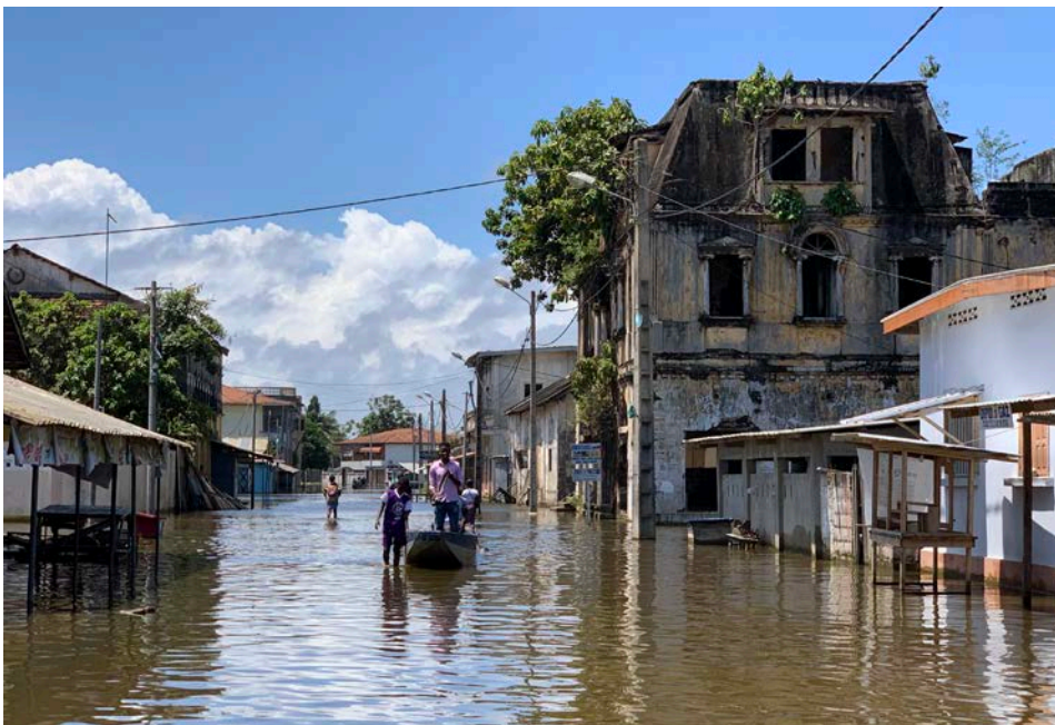
Heavy rain led to severe flooding across the World Heritage Site of the 'Historic Town of Grand-Bassam', October 2019. ©UNESCO
