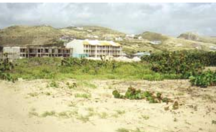
New hotel under construction at Frigate Bay, St Kitts, 2000, well inland from the active beach zone and the seaward dune – an example of good stewardship.
