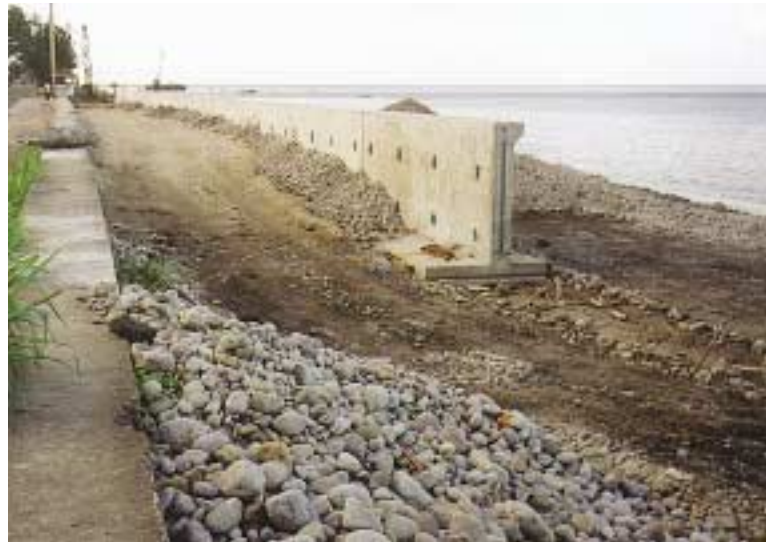
New seawall under construction, Pottersville, Dominica. 2001.
