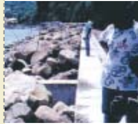
Hard engineering structures, such as this rock revetment at Victoria, Grenada, serve to protect the land, in this case, the coastal highway from erosion; but they do not promote the build-up of sand, 1999
