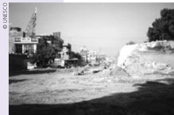
375 years old hydraulic works (on the right), demolished due to urban pressure, Lahore Fort, Pakistan
