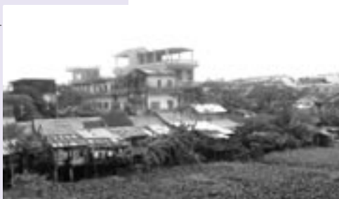
Illegal constructions marring the traditional skyline of the Citadel of Hue, Vietnam
