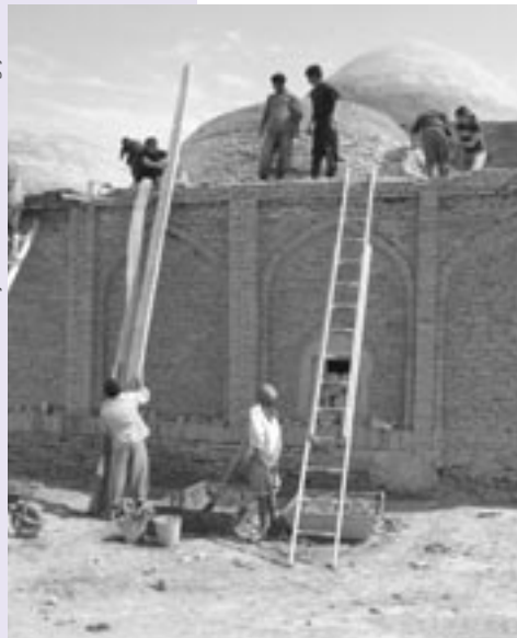
Restoration work at Ibn Zayd, Ancient Merv, Turkmenistan
