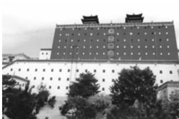
The Red Terrace of Putuozongchenshimiao after renovation, Chengde Mountain Resort, China
