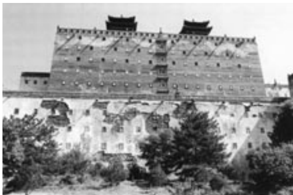
The Red Terrace of Putuozongchenshimiao before renovation, Chengde Mountain Resort, China
