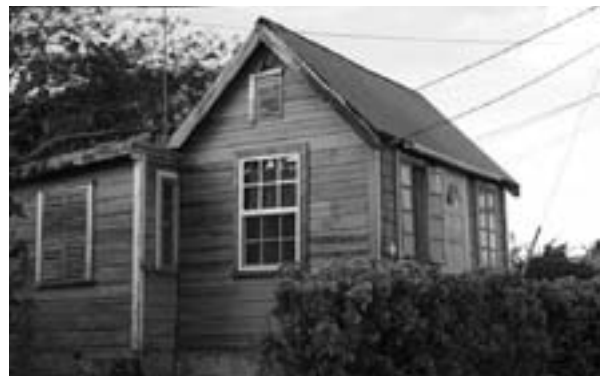
A chattel house in design transition, where there are varying window types: jalousie, sash and double-hung glass. The entrance door is also on the move.
