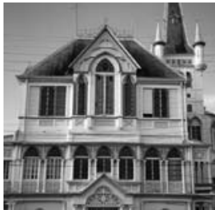
Georgetown's City Hall: an extraordinary example of Gothic architecture in a tropical context, executed in wood with cast-iron elements
