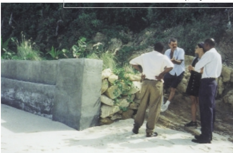
Group of planners and developers discussing a recently constructed seawall at Meads Bay, Anguilla, 1998
