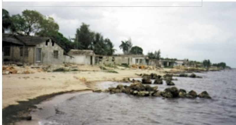
Groynes built by the community to promote beach accretion and protect houses at Playa Mayabeque, Helena del Sur, Cuba, 2001
