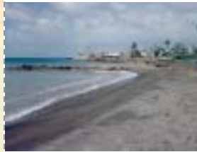
(below) Groynes, such as seen here at Sugar Bay in 1989, result in sand build-up on one side, but erosion on the other side
