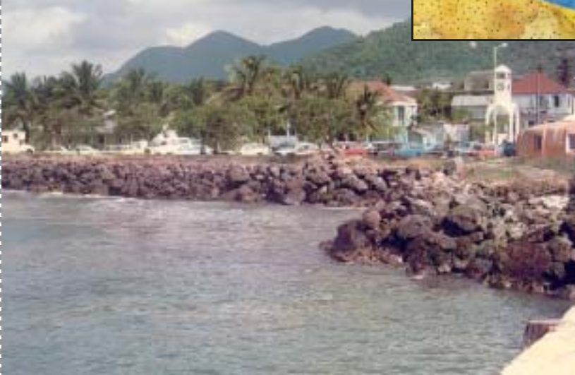
(below) Groynes, such as seen here at Sugar Bay in 1989, result in sand build-up on one side, but erosion on the other side
