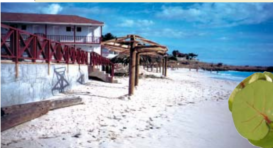
Vertical retaining walls protect properties but do not promote beach build-up, Crab Hill Bay, Antigua, 2000
