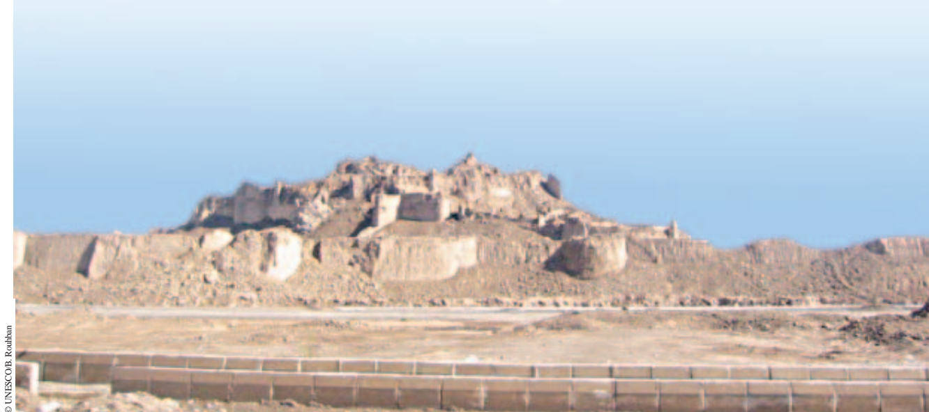
The badly damaged Bam Citadel (Arg-e-Bam)
