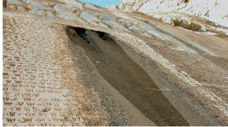
Algae and lichen around seepage water.
