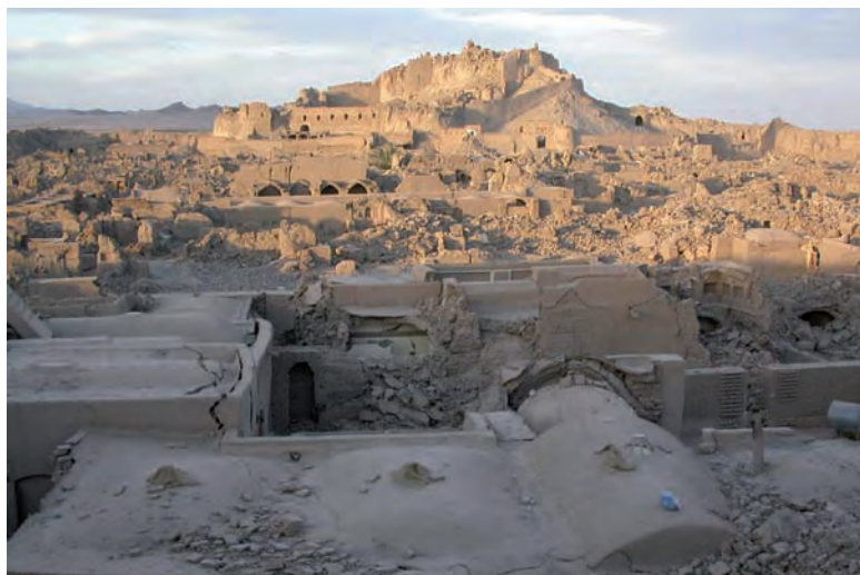
Damage to Bam and its Cultural Landscape (Islamic Republic of Iran) caused by an earthquake.
