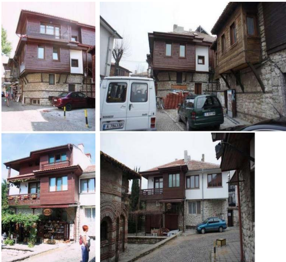
Examples of the removal of illegal additions to buildings within the historic town. Left: the buildings with illegal additions as they were before; right: the buildings after the removal of the illegal extensions. (© Images provided by the State Party)
