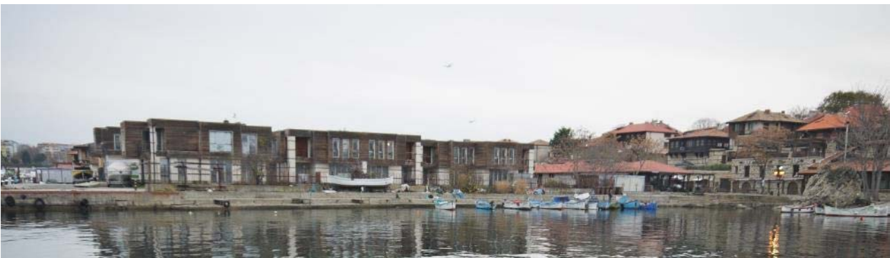
Planning permission was granted for construction next to the Marina on the basis that the project conforms to requirements for the buffer zone, e.g. height restrictions, but no formal assessment of the impact of this project on OUV seems to have taken place. (© Sarah Court/ICOMOS)
