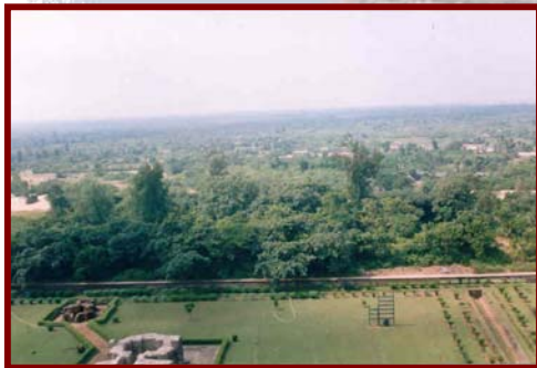
← AERIAL VIEW WEST SIDE
