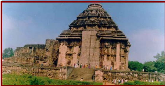
GENERAL VIEW, SOUTH SIDE
