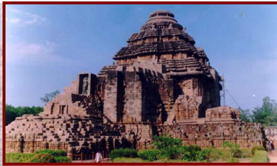
GENERAL VIEW, WEST SIDE
