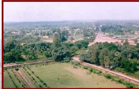
AERIAL VIEW NORTH-WEST SIDE →
