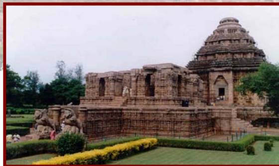
GENERAL VIEW, EAST SIDE
