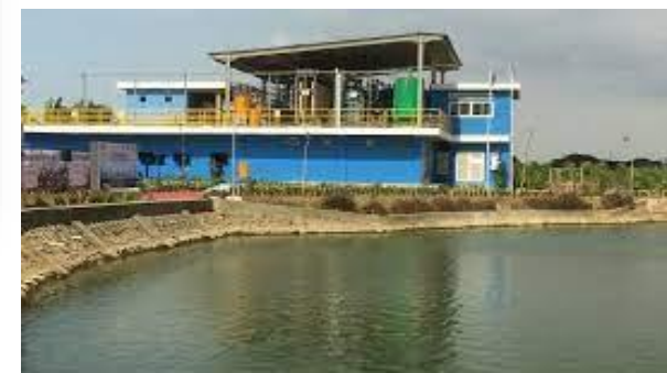
Central of clean water treatment
