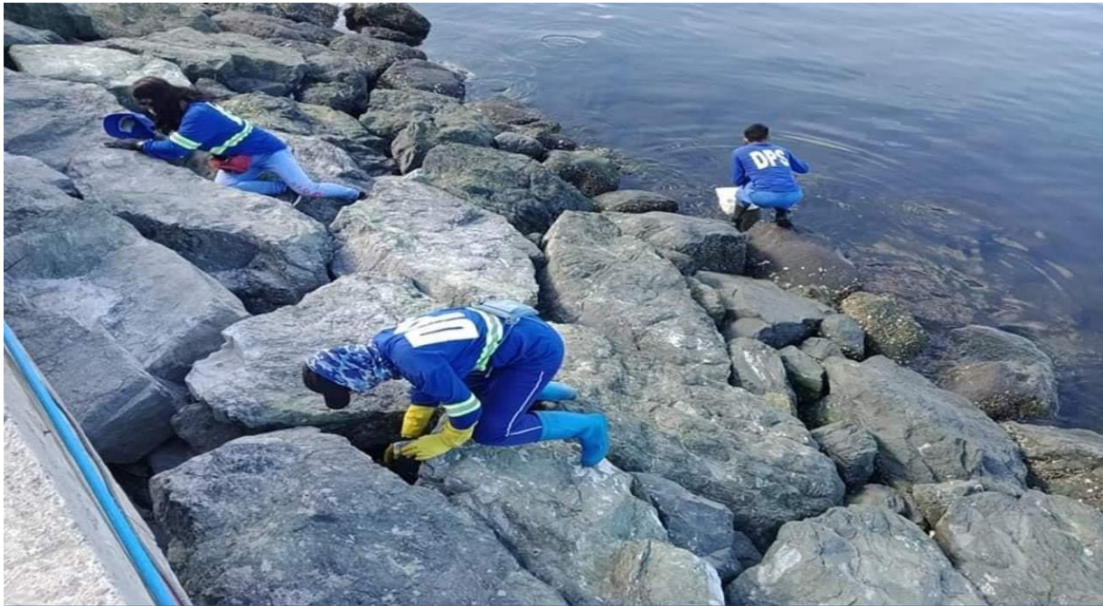
Location: Baywalk, Manila Yacht Club, Dist. 5 Date: March 3, 2021 Truckloads: 1/4 (Shacman)
