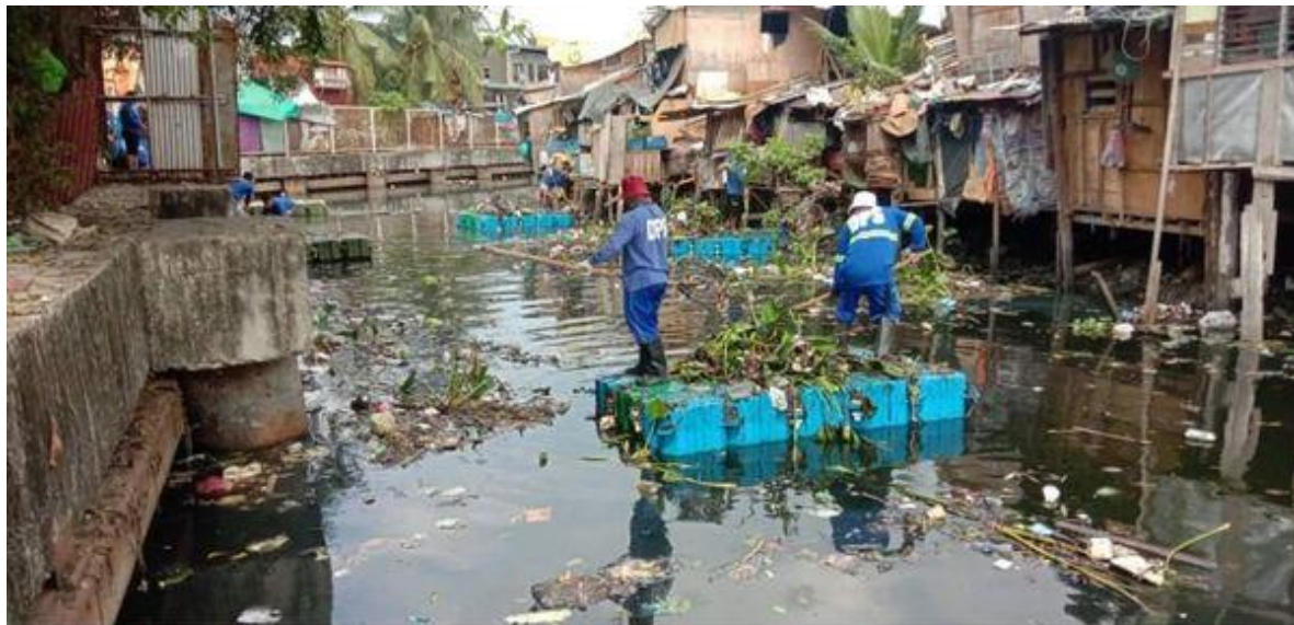
Location: Estero De Sunog Apog Brgy. 135 Zone 12 District I Date: March 1, 2021
