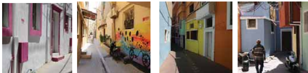
■ The walls of the residential facades in the southern quarter of the old city were cleaned and painted and the electricity wiring were arranged properly to avoid visual pollution.
