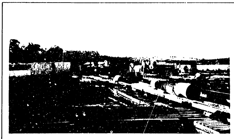
FIGURE 13: THE FLOATING NET-CAGE SYSTEM CONSISTS OF THE NET-CAGE PROPER AND A WOODEN RAFT TO SUPPORT THE NETS. NEXT TO THE PLATFORM SUPPORTING THE CAGES IS A MAIN HOUSE-CUM-OFFICE, WHICH OPENS ONTO THE SHADED WORKING AND EQUIPMENT STORAGE AREA
