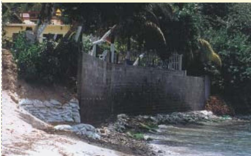
*Vertical walls, such as here at South Frigate Bay, interfere with natural beach processes, 1995*
