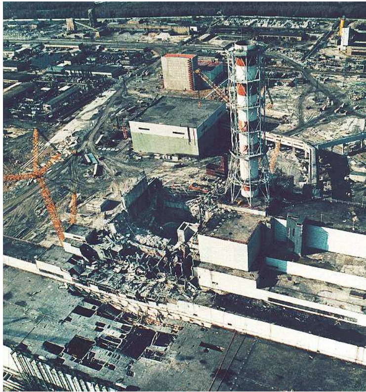
Aerial view of destroyed Chernobyl reactor after the accident in 1986 showing the extent of the damage caused. Photo: European Bank for Reconstruction and Development.
