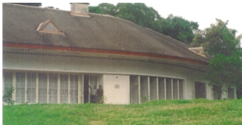
Known affectionately to students as 'ERAIFT Castle', the school building dominates the valley with a breathtaking view of Kinshasa and the Congo River in the distance
