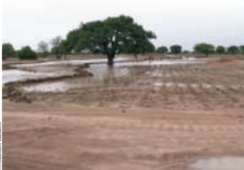
Rainwater harvesting in Burkina Faso using low-cost hand-constructed structures
