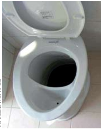
This eco-san toilet separates faeces (back) and urine (front) into two distinct compartments, making the treatment of waste easier and less costly. Studies have shown that the nutrients from human urine can be used to grow enough food to feed a person for a day
