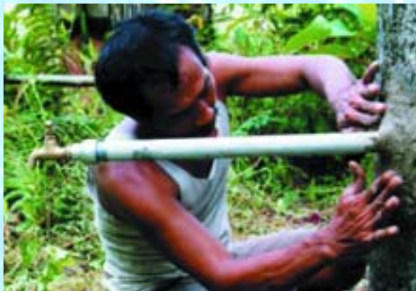
A local man fixes the tap onto the water tank
