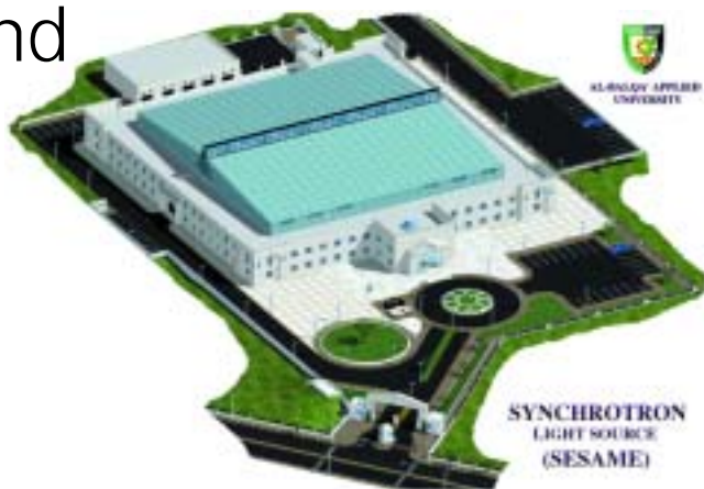
The future SESAME building
