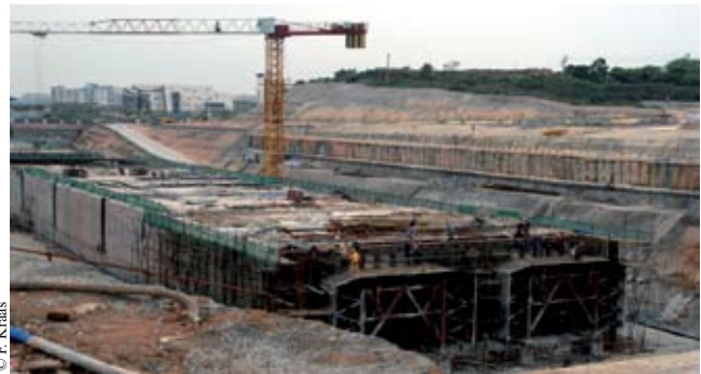
Construction of the Guangzhou underground railway system in China in March 2008
