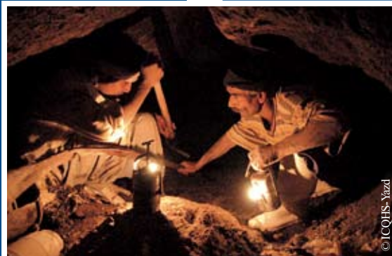
Workmen repairing one of Bam's qanats
