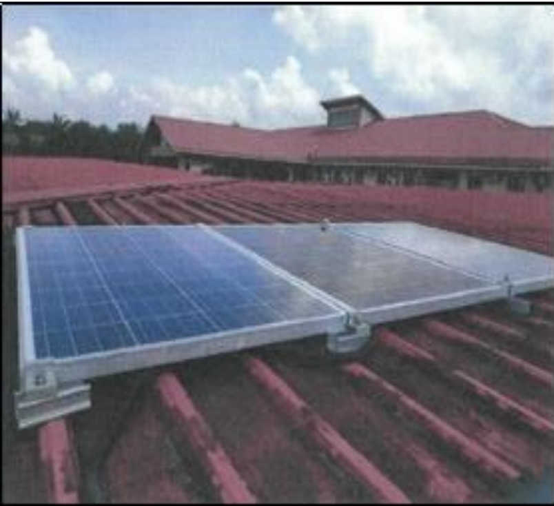
Installation of solar panel
