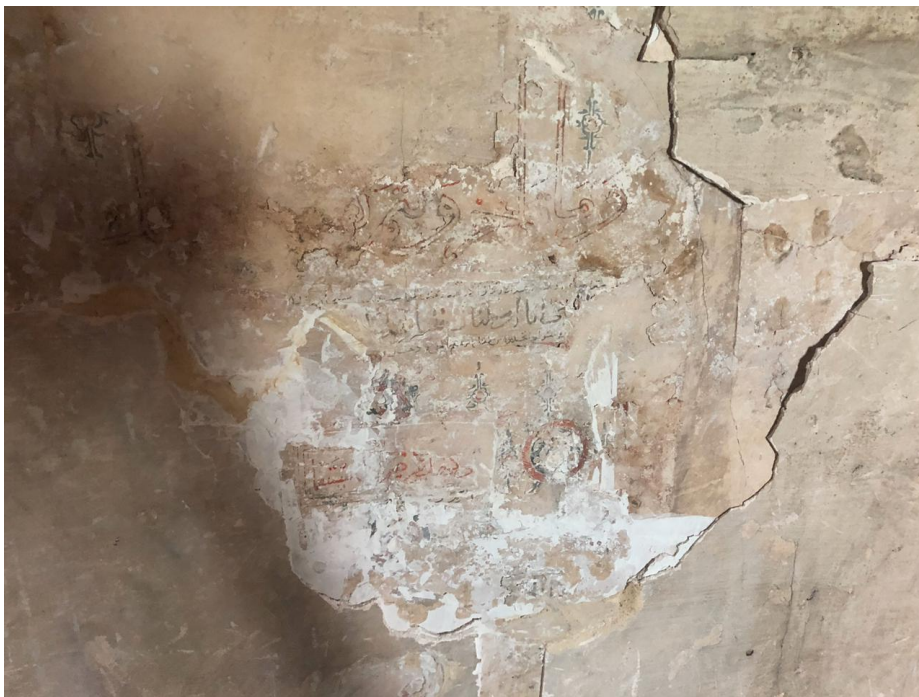
Image 2: an Example of the written text behind the new plaster layer on the wall of the Qibla, © EHRF.
