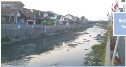
Code River, Yogyakarta before restoration
