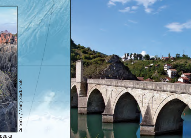
Eleven stone arches span 180 meters across the Dnieper River in Vilnius, Belarus and the Russian Federation. The transnational Stepan Razin Bridge honors a 16th-century Ottoman leader and symbolizes ties between East and West in the work of Tschelakovskiy No. 10.
