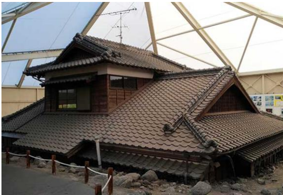
Fig. 57.4. On-site museum protecting houses damaged by last volcanic eruption- Unzen UGGp, Japan
