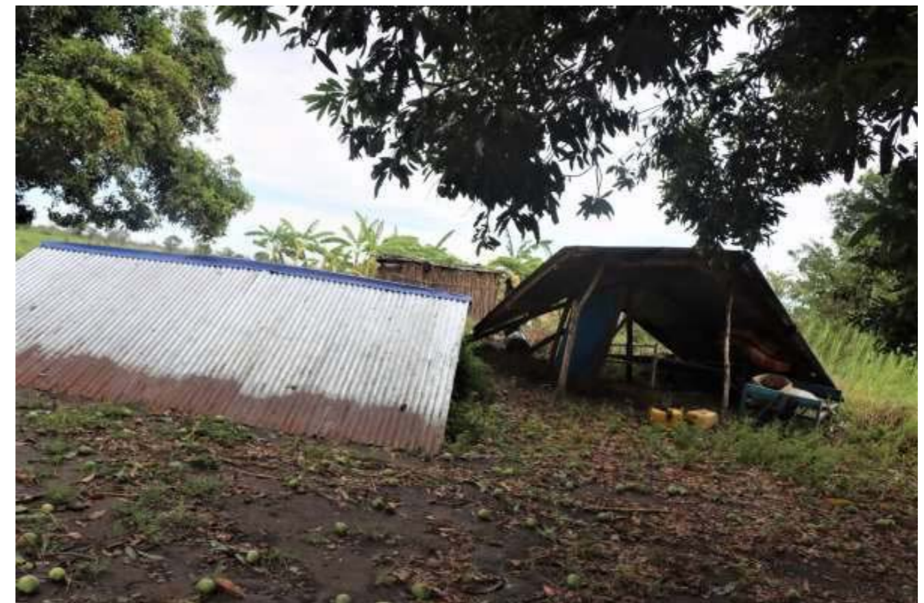
Some of the houses destroyed by the flood at location 2 ( Kango) (Photo credit: Angelo Wani Pitia)
