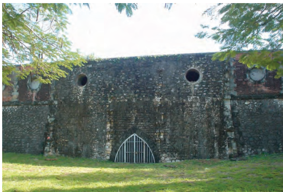
Water Reservoir, Nouméa, New Caledonia.
