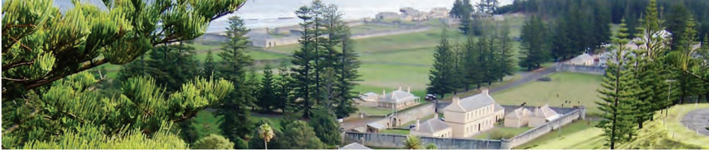
Administrative and Military settlement along Quality Row overlooking the Prisoners Compounds and Pier Precinct along the water front. Reproduced courtesy of: KAVHA Management Board
