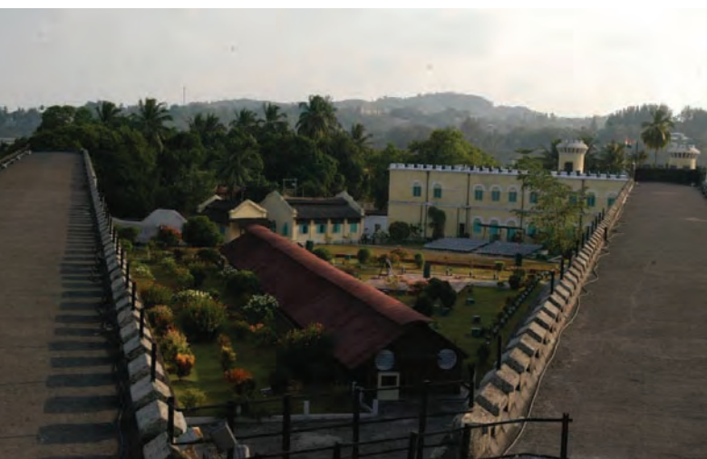
Panopticon design radial wings of Cellular Jail, Andaman Islands.
