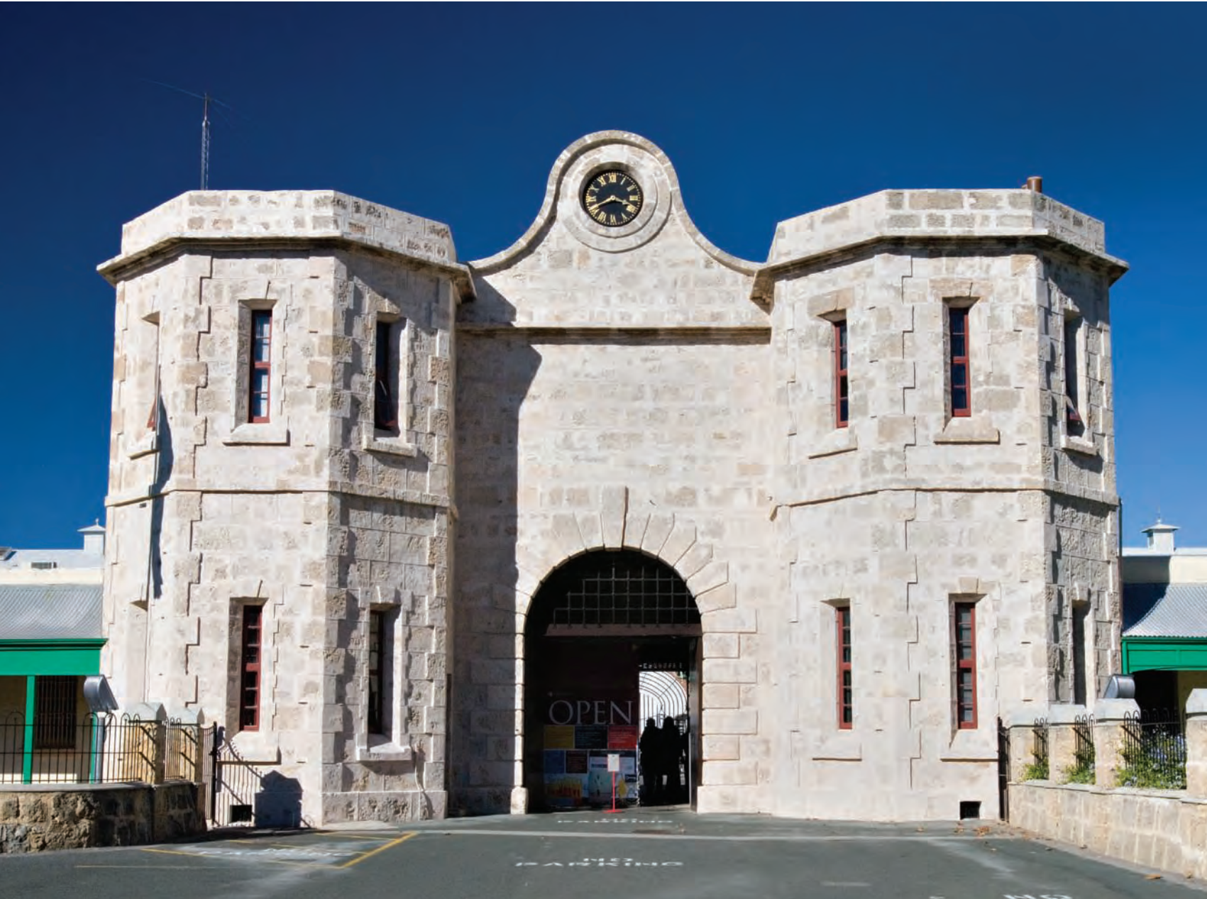
Fortified Gatehouse entrance to the prison.
