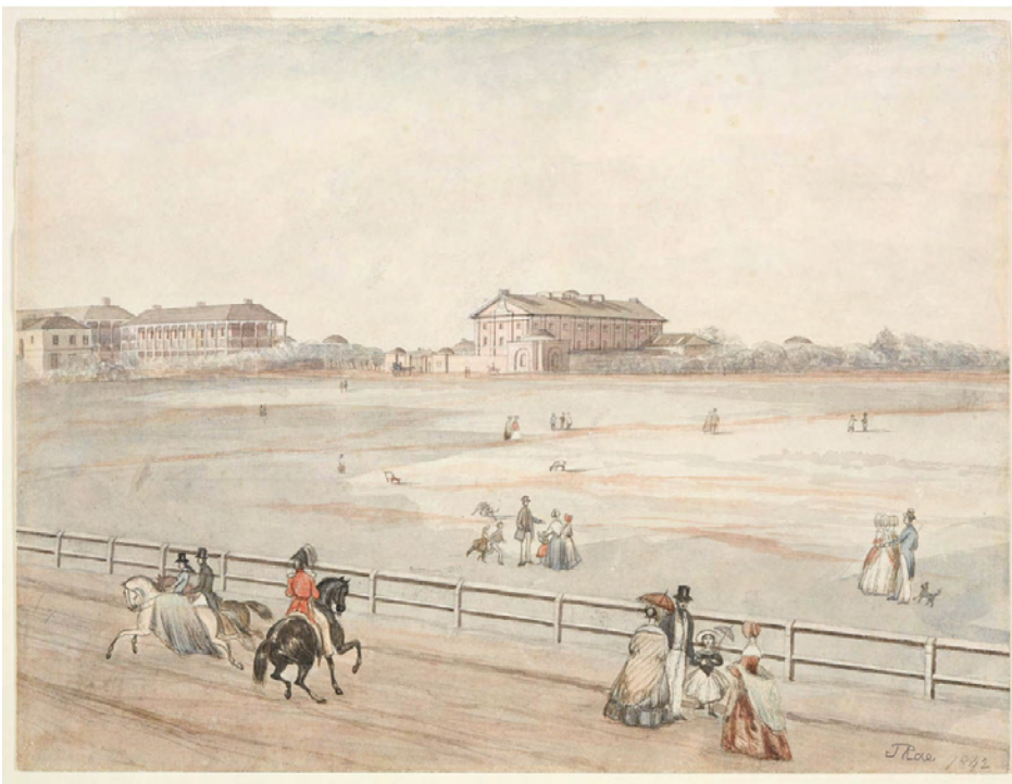
Figure 8: View of Hyde Park Barracks, looking eastwards across Hyde Park North from Elizabeth Street, watercolour by John Rae, c1842. The two-storied building on the left is the southern wing of the General, or Rum, Hospital.
