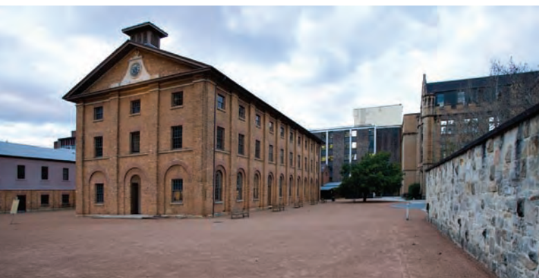
Hyde Park Barracks showing the external building, the area convicts were mustered and the perimeter wall.
