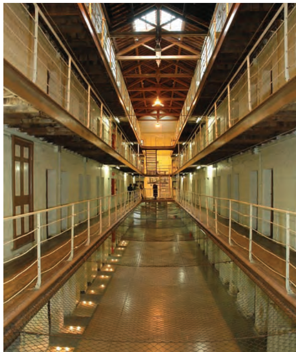
Interior of one wing showing elements of Pentonville design with front facing cells along galleried walkways.
