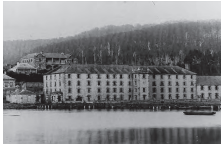
Historical photograph of the four-storey Penitentiary.
