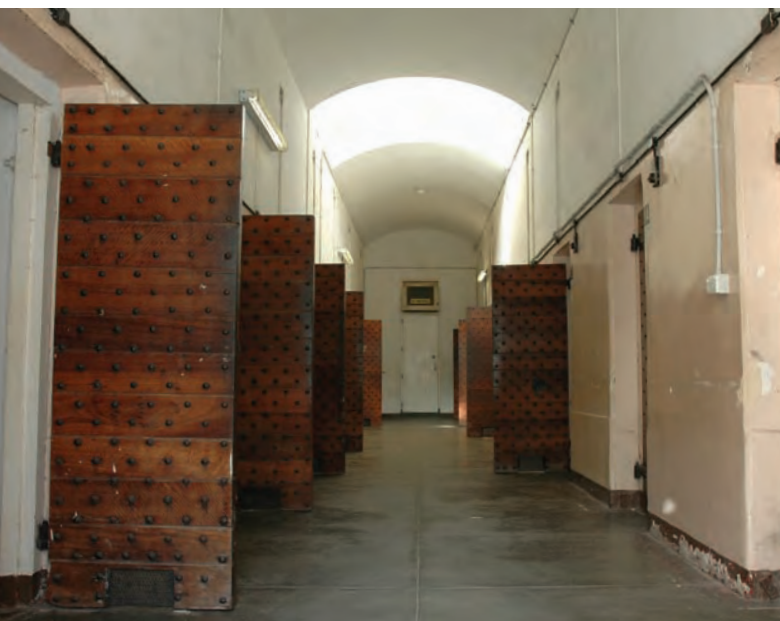
Solitary confinement cells in the Refractory Cell Block for unruly convicts.
