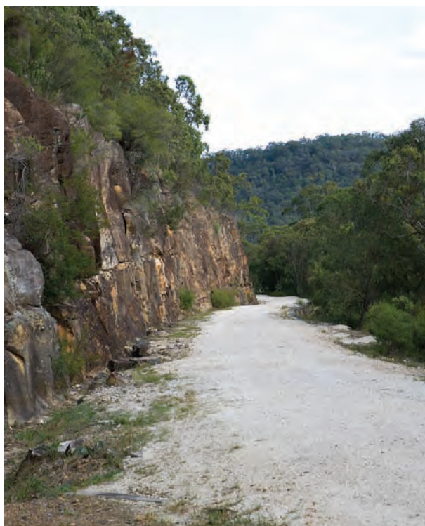
Old Great North Road's original setting has a strong sense of place and character from the convict days.
