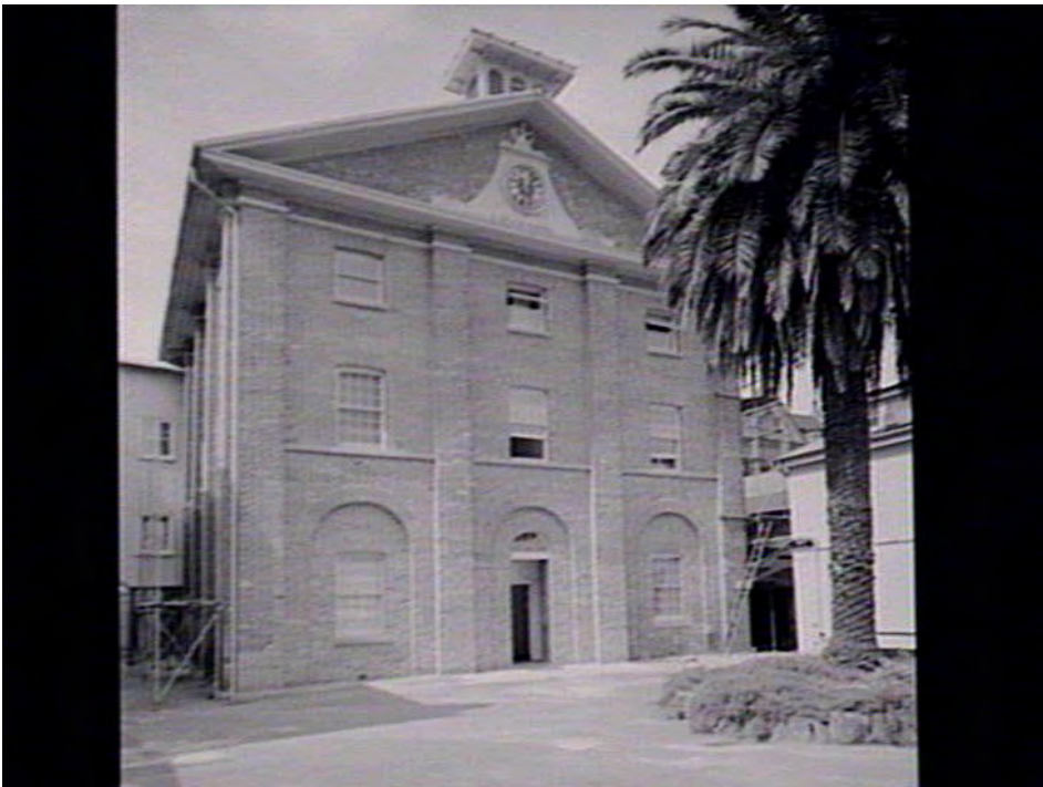
Figure 10: View of Hyde Park Barracks during first phase of works to remove Court structures and convert to a museum use in 1976. Source:
