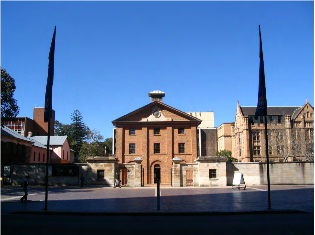
Figure 15: current condition of the site – Façade of the brick central Barracks building, with stone gateway and western perimeter wall, and brick northern range of buildings on left, all in good to very good condition.
