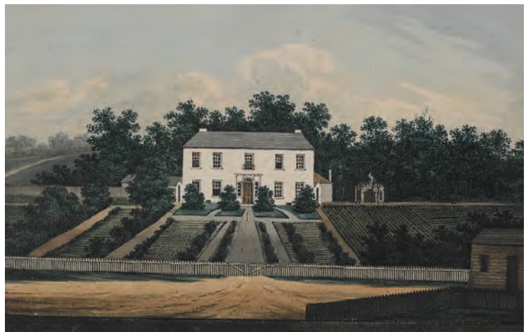
A view of the Government House at Parramatta in 1805 before the Governor Macquarie extensions.
