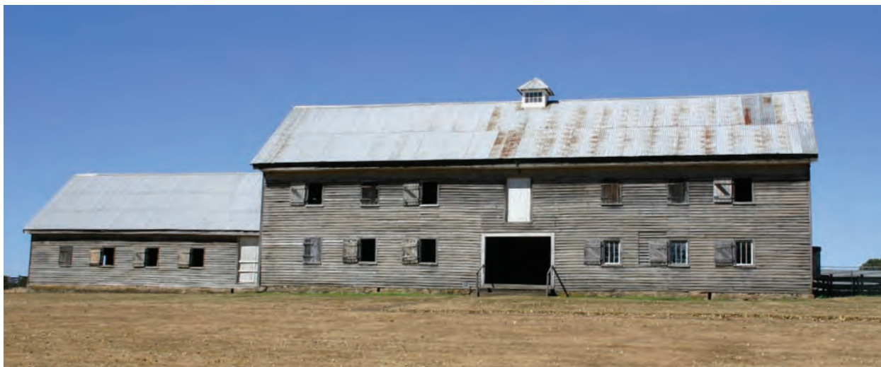
Cider House (left) and Woolshed (right) at Woolmers Estate where convicts laboured under the assignment system.
