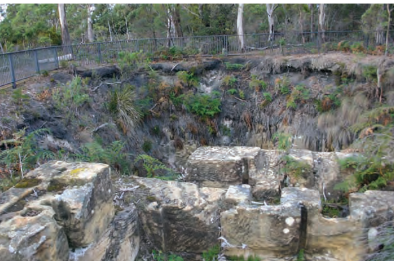
Opening of the main coal shaft where convicts laboured in stifling underground conditions.
