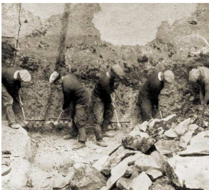
Stone-working is an important part of the history of the Site at Beer, Purbeck and on the Isle of Portland. This picture from Portland shows a group of workers splitting the stone by hand using hammers and wedges.
