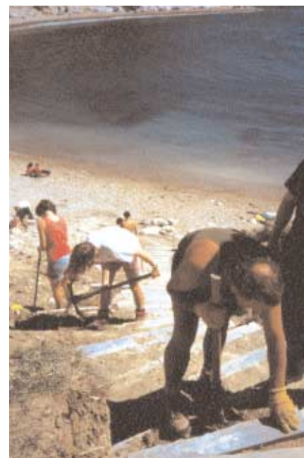
Regular maintenance of heavily used paths is required. This group of volunteers is repairing access steps at Man o'War Bay.
