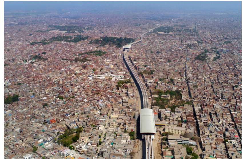
Orange Line Metro Lahore Picture Credit: Habib Construction Services
