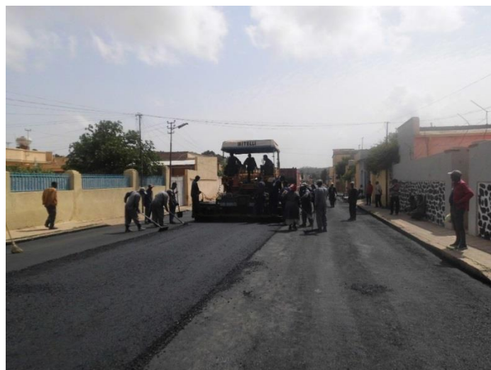
Ge'za Banda neighborhood under road infrastructure overlaying maintenance activity, April- May 2020
