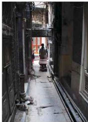
Above: Koocha Charkh Garan, before and after rehabilitation
