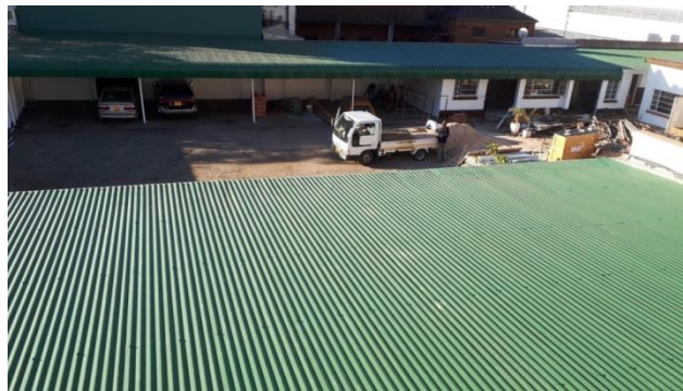
New roof on Douslin House
