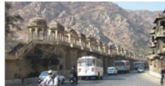
National Highway diverted to save cultural landscape and 52 heritage properties. Ghat ki Guni, Jaipur (Source:Dronah)
