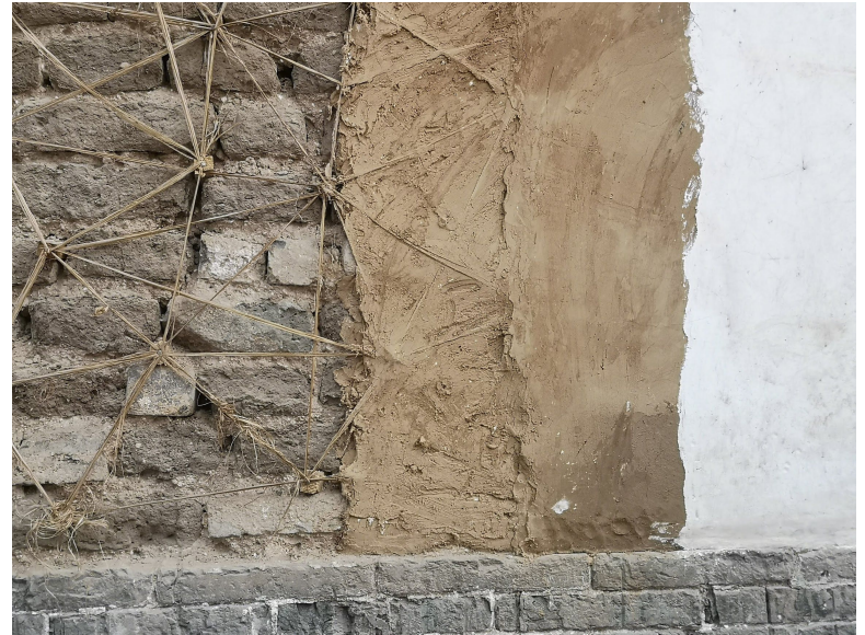
Traditional conservation plaster application in houses in Jinan, China (Source: SJ)
