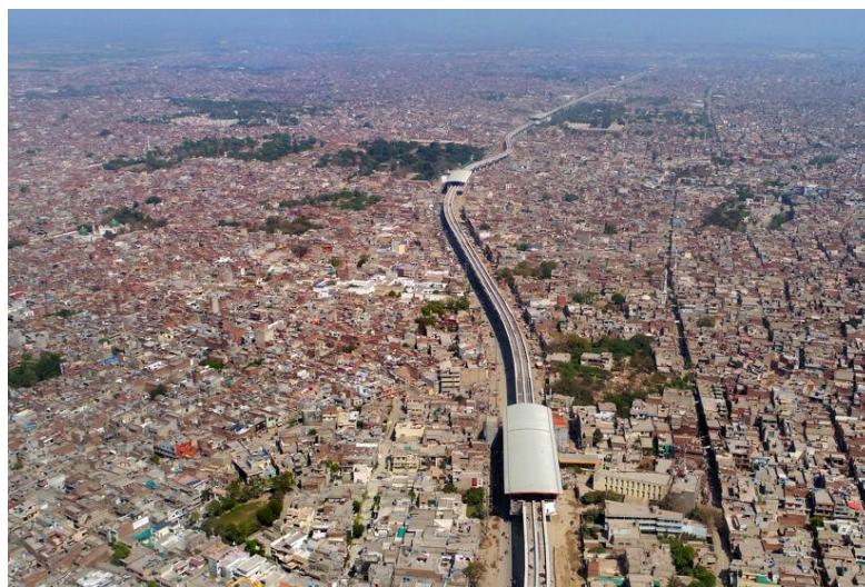
Orange Line Metro Lahore Picture Credit: Habib Construction Services
