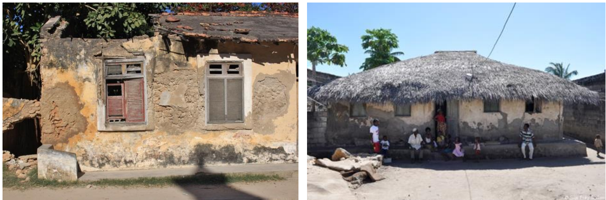
Dilapidated houses in Macuti
