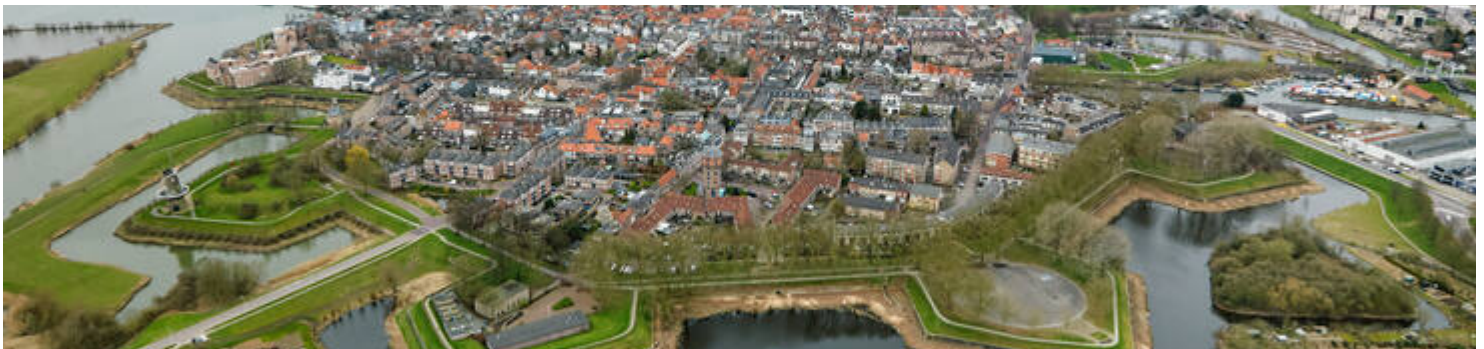
Dutch Water Defence Lines (extension of the Defence Line of Amsterdam). Fortified town of Gorinchem © New Dutch Waterline
