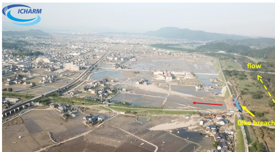
Fig. 1 Levee breach and inundation in Mabi Town (photo by ICHARM, July 2018).
